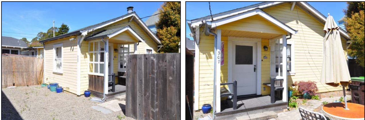
Figures 2 and 3. Left image shows the front (east) and south elevations. Note the metal chimney and porch modifications. The earlier, rear section is located behind the fence. Right image details the front elevation.
