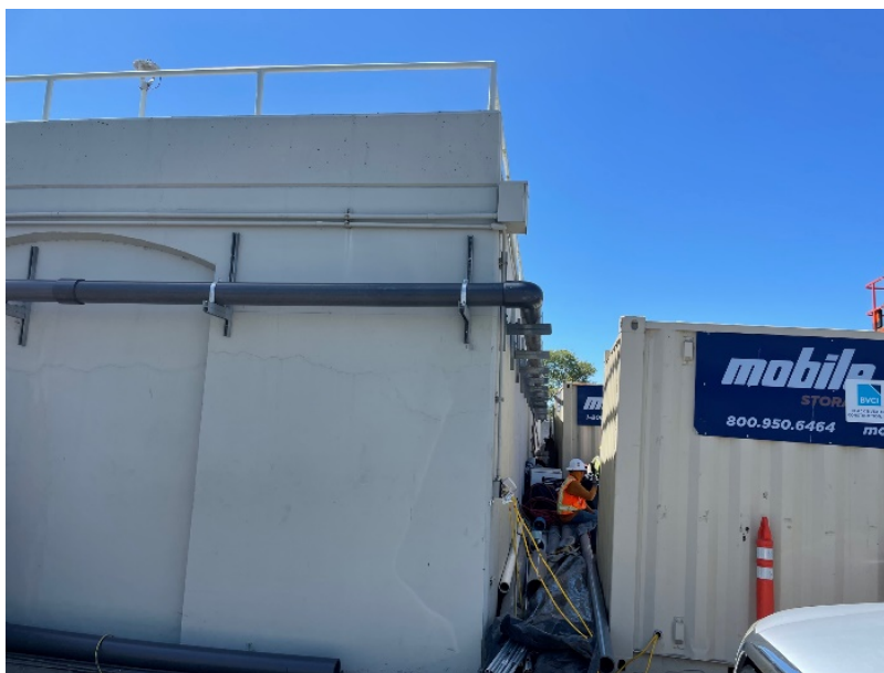
New 6" tertiary treated pipeline braced to existing structure
