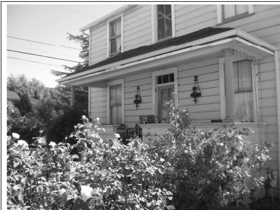
Photo 2: View of the front porch and entry.
