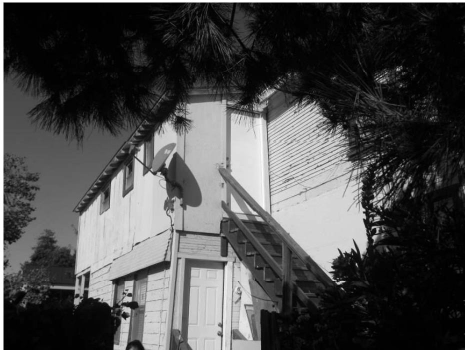
Photo 9: Another view of the rear entries.
