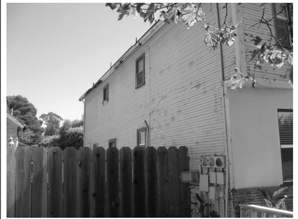
Photo 5: View along the northern façade.
