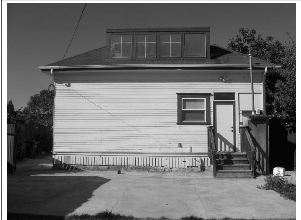
Photo 7: View of the rear façade.
