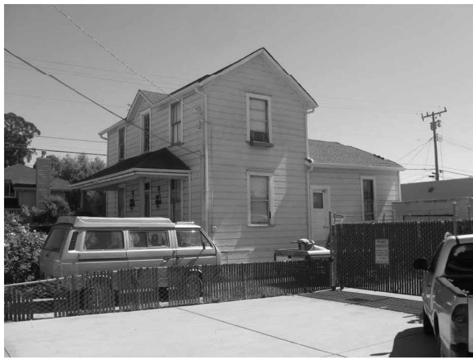
Photo 3: Oblique view of the residence from the northwest.
