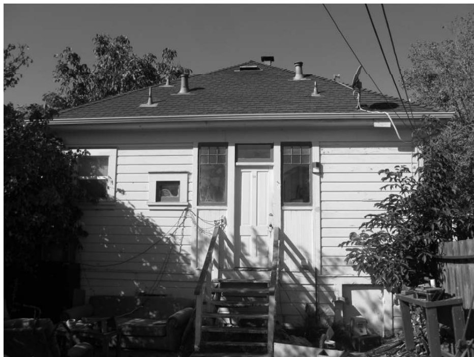
Photo 9: View of the rear of the structure.
