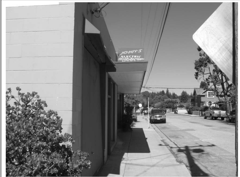
Photo 7: View along the front façade showing awning and sign.
