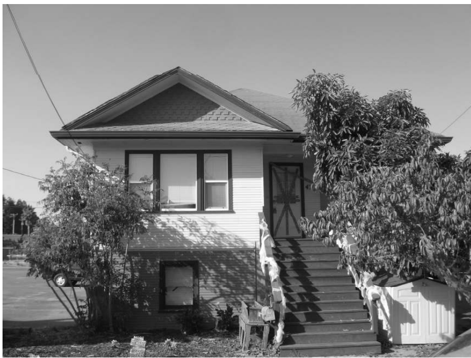
Photo 1: View of the front façade of 431 May Avenue
