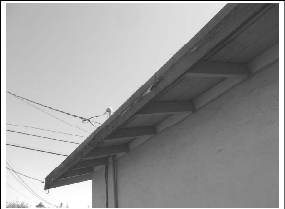
Photo 4: View of the broad eaves with exposed rafters.
