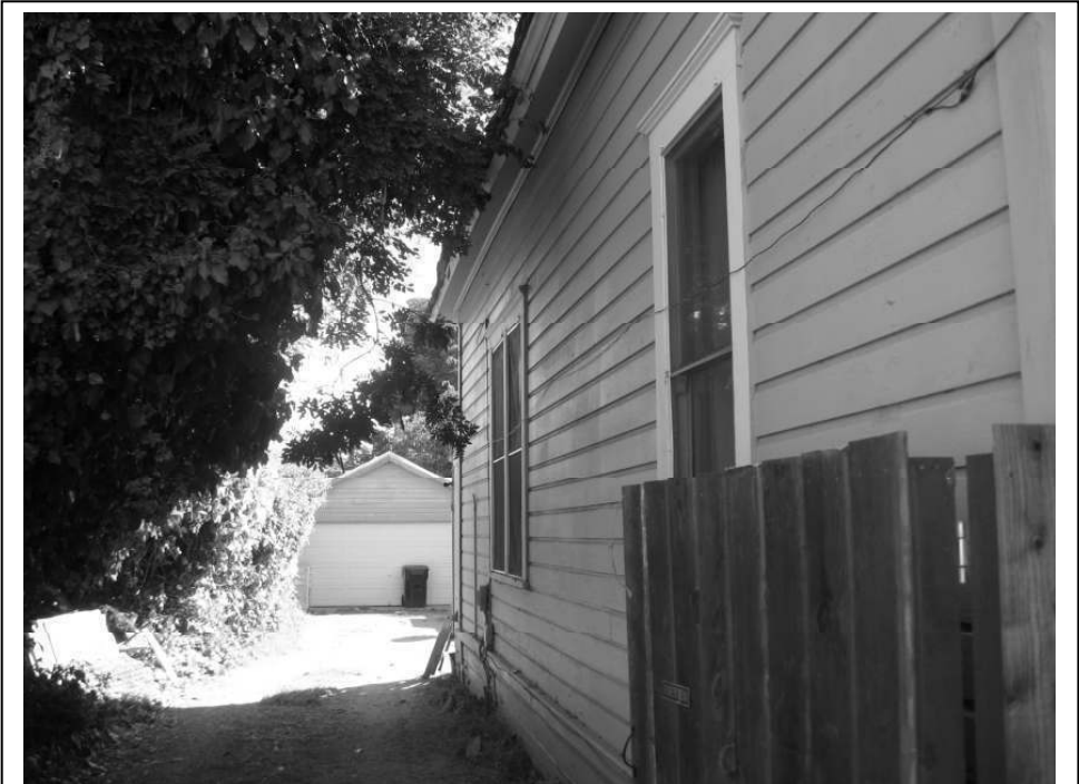
Photo 8: View along the northern façade.
