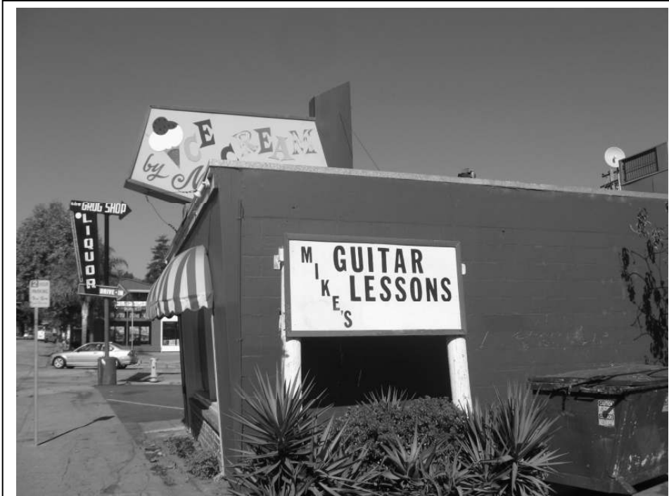
Photo 7: View of the front portion of the southern façade.
