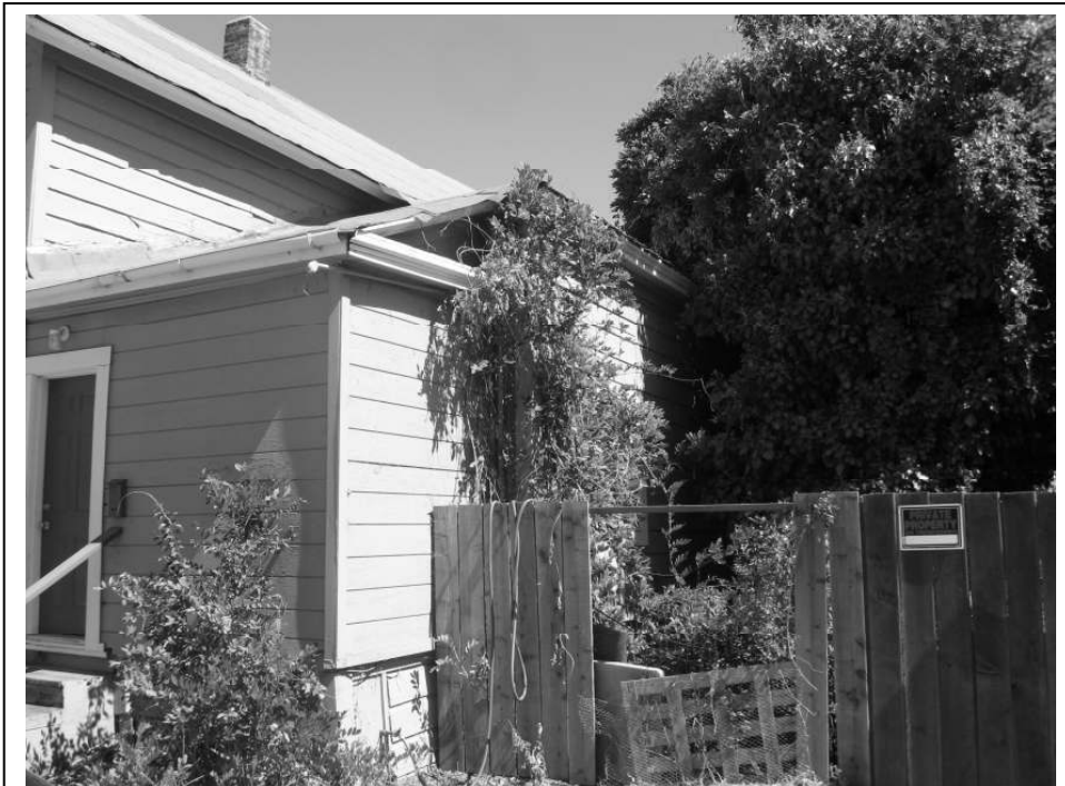
Photo 6: View along the southern façade showing southern wing.
