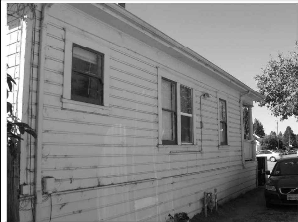
Photo 7: View along the northern façade from the east.
