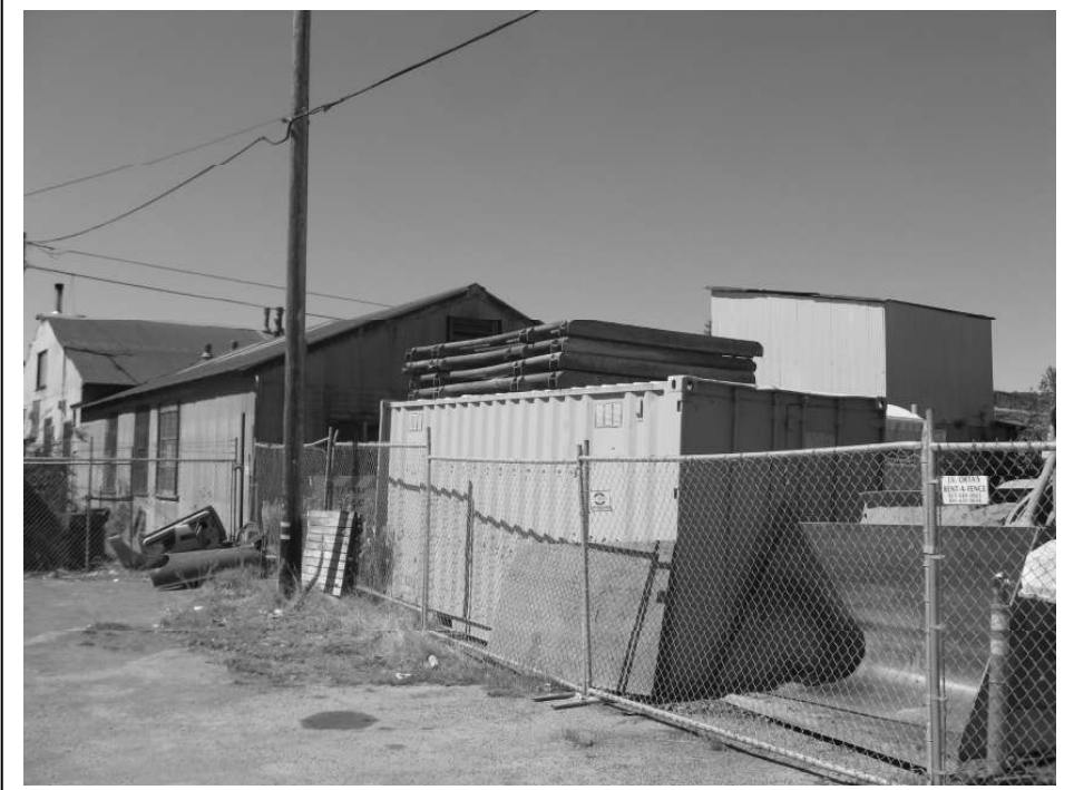
Photo 9: View of the southern portion of the rear façade.
