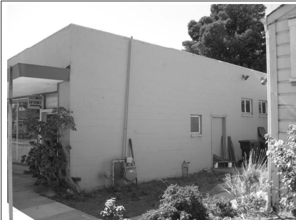
Photo 4: View of the northern façade of the structure.
