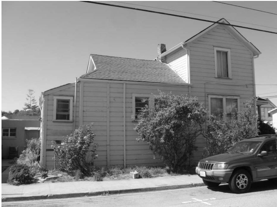
Photo 5: View of the eastern façade showing both rear additions.
