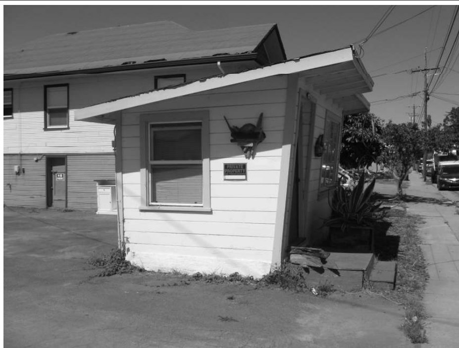
Photo 10: View of 429 May Avenue from the south.
