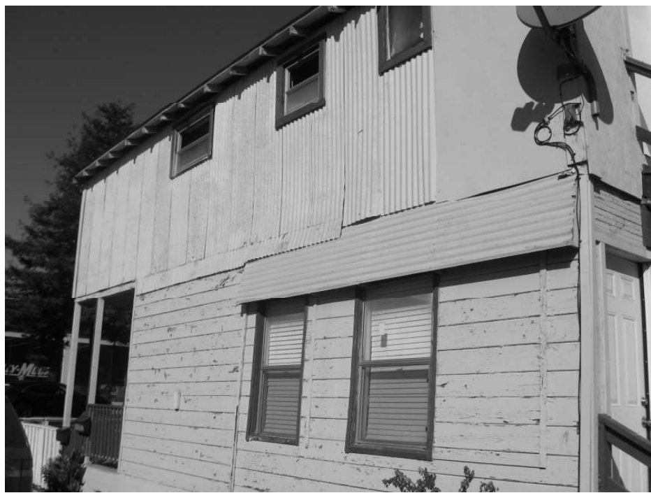
Photo 7: View of the side addition from the south.
