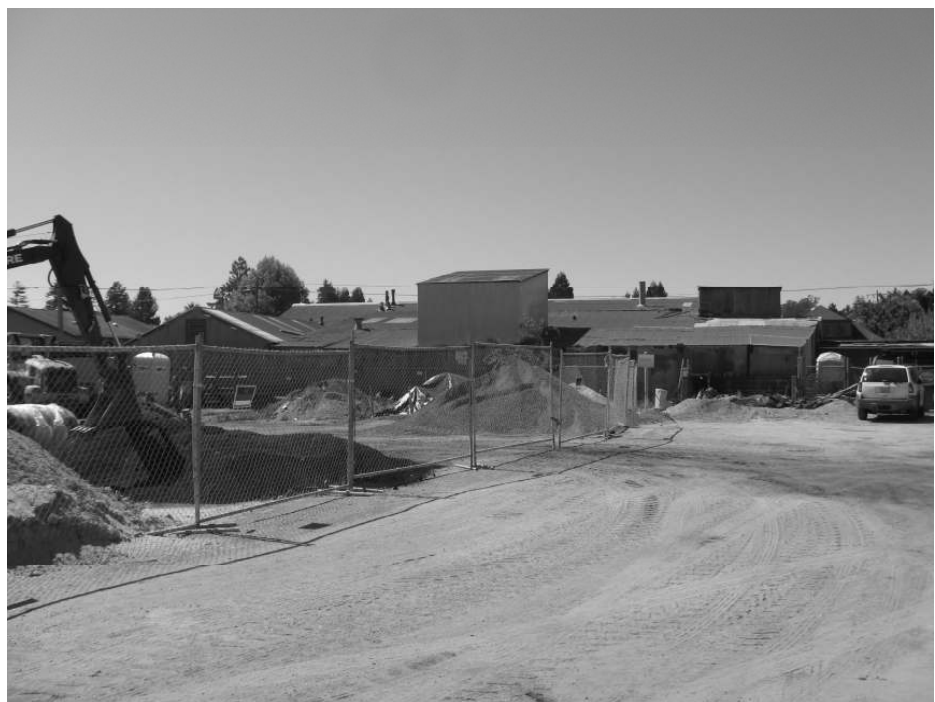
Photo 8: View of the rear façade.
