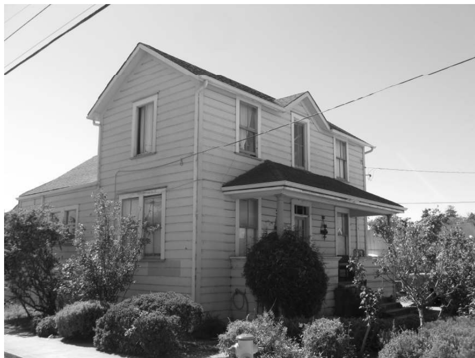
Photo 4: Oblique view of the residence from the northeast.
