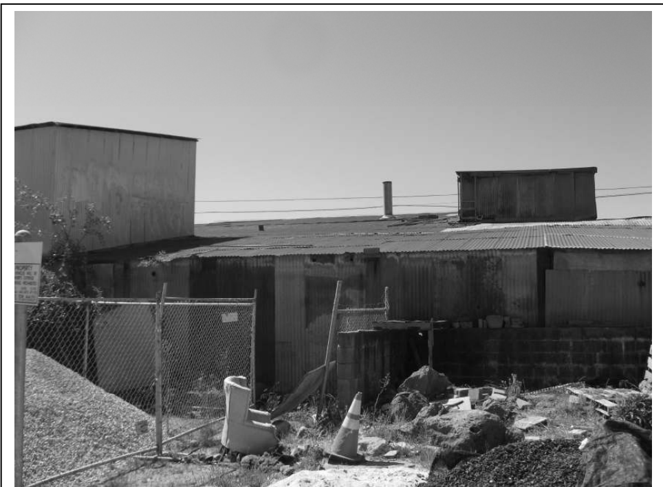
Photo 10: View of the northern portion of the rear façade.
