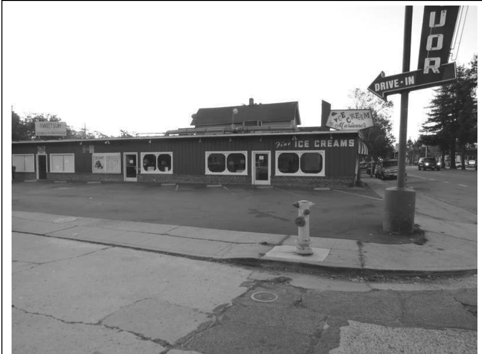
Photo 3: View of the western façade from Ocean Street.
