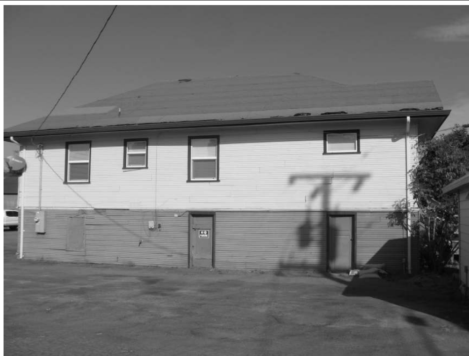
Photo 6: View of the southern façade of the residence.
