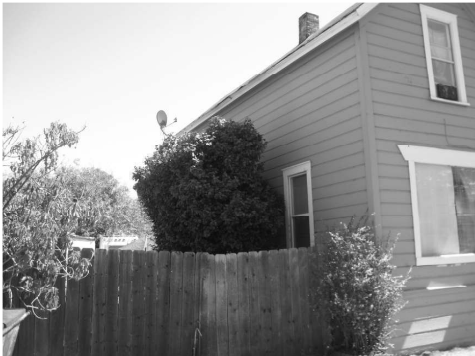
Photo 4: View along the northern façade of the residence.
