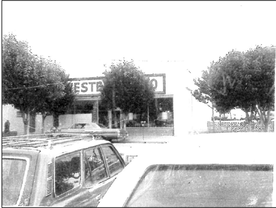
Figure 6. 1974 Santa Cruz County Assessor’s photograph of the front (north) elevation. Note the earlier storefront and Western Auto sign.
