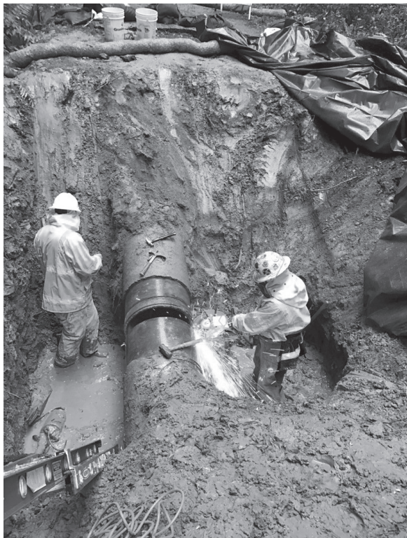
Workers repair 2017 storm damage to the water system
