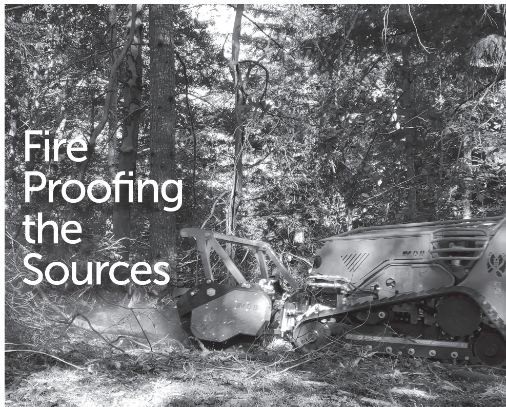
A Water Department team uses a masticator to reduce fire fuels in the Newell Creek watershed
