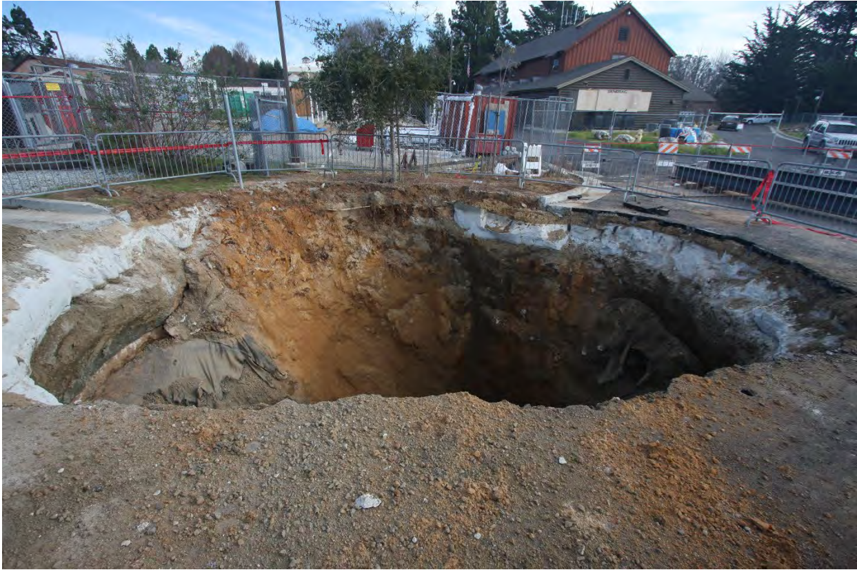
Figure 1 - 2015 photo of sinkhole developed within a reactivated doline under a stormwater treatment system on the UCSC campus
