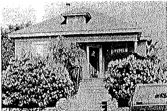
424 Mott Avenue Colonial Revival 1895-1915
