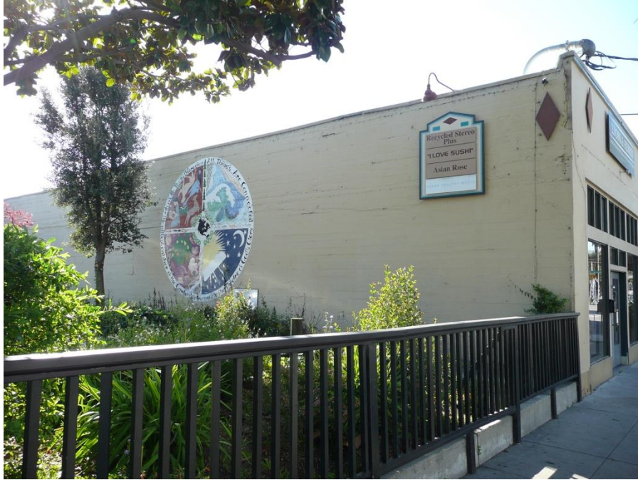
Figure 24: The western portion of the north elevation of the 1926 building, facing southeast.
