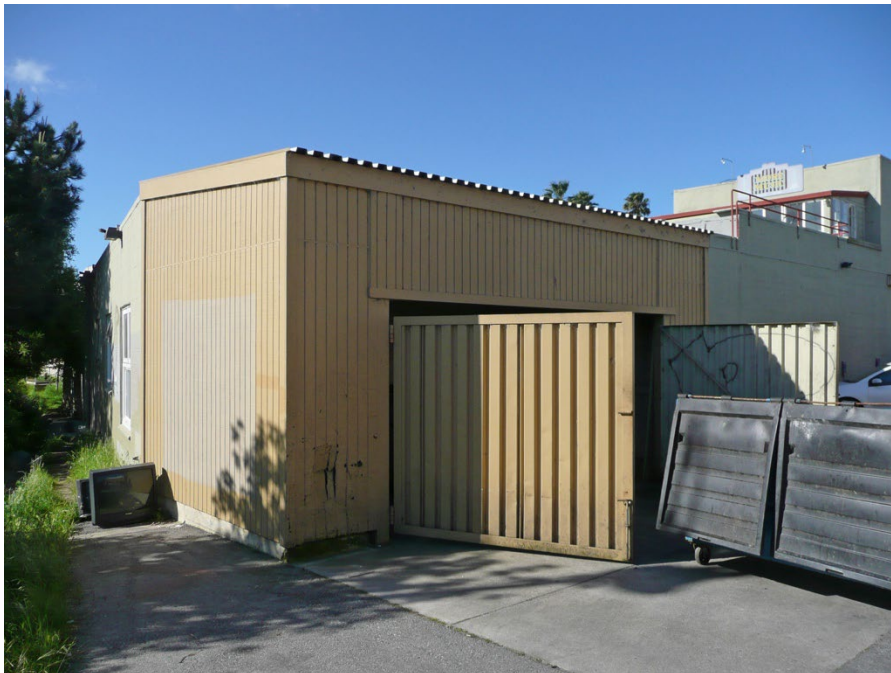
East and north elevations of the ca. 2007 Shed 1, with the neighboring building at 512 Front Street visible at left and right of the ca. 2007 Shed 1, facing southwest.
