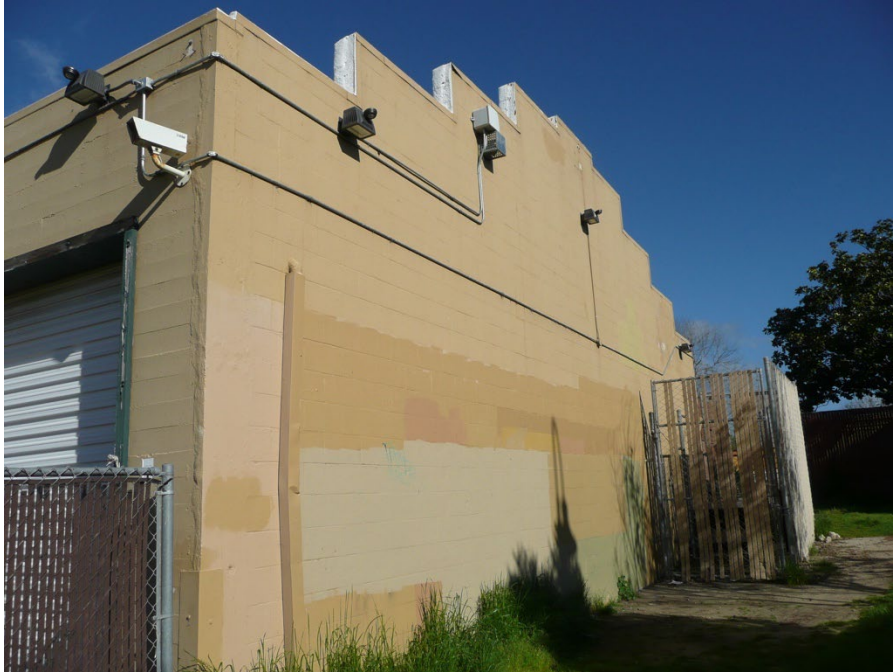
East elevation of the rear wing, facing north-northwest.
