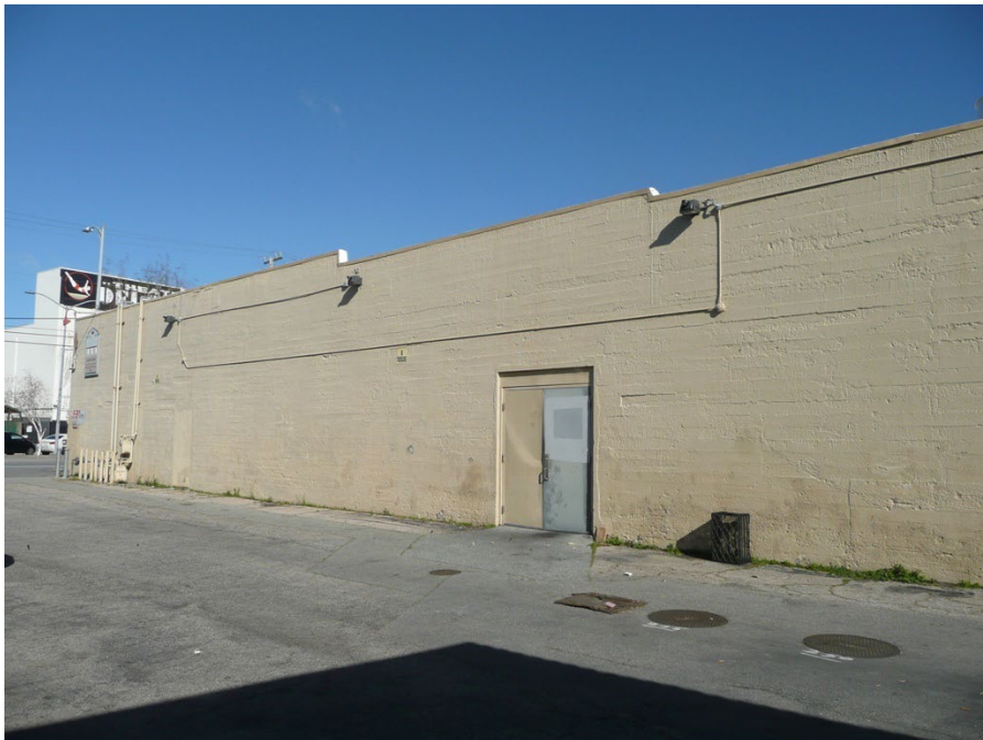
South elevation of the 1926 building, facing northwest.
