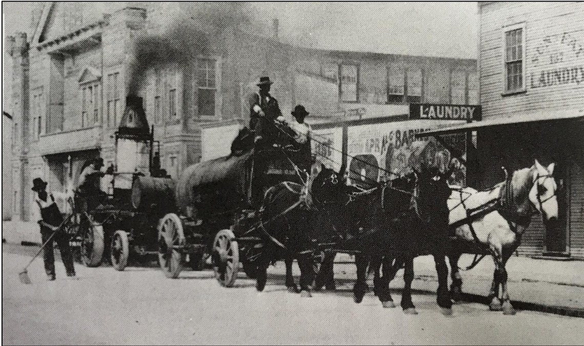
Figure 6: ca. 1900 photograph of the buildings that existed on the subject parcel prior to the construction of the 1926 building—situated between the Armory building at left and the Sun Fat Laundry at right. (Photo from Santa Cruz County: Parade of the Past by Margaret Koch)
