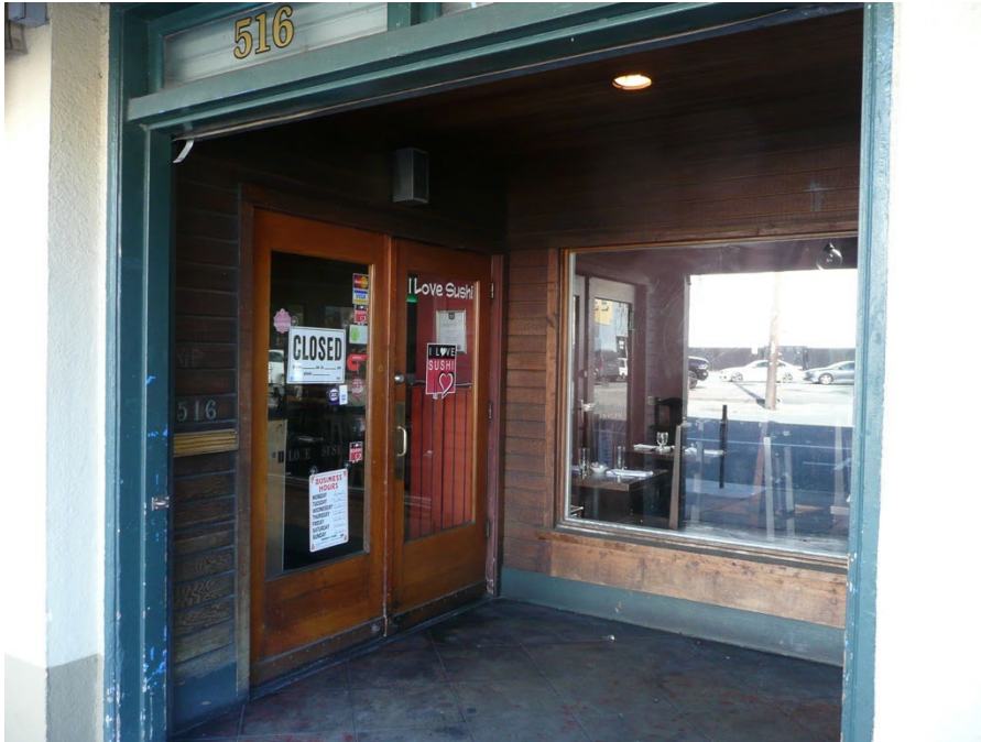
Detail of recessed opening within the center bay, showing the south-facing double doors and plate-glass window, facing northeast.
