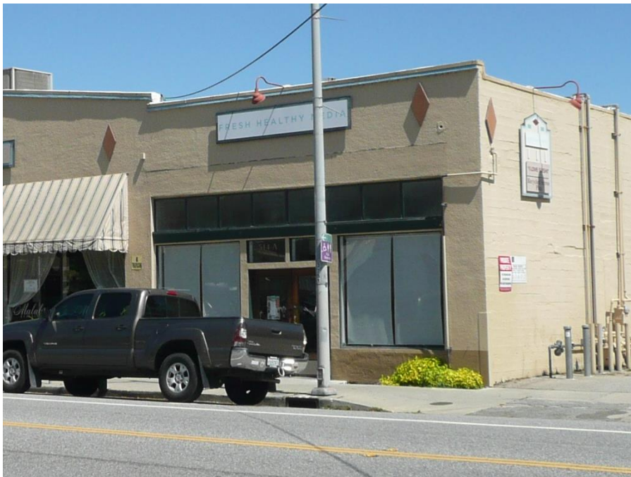
Figure 13: The west elevation at the southernmost bay, facing northeast.
