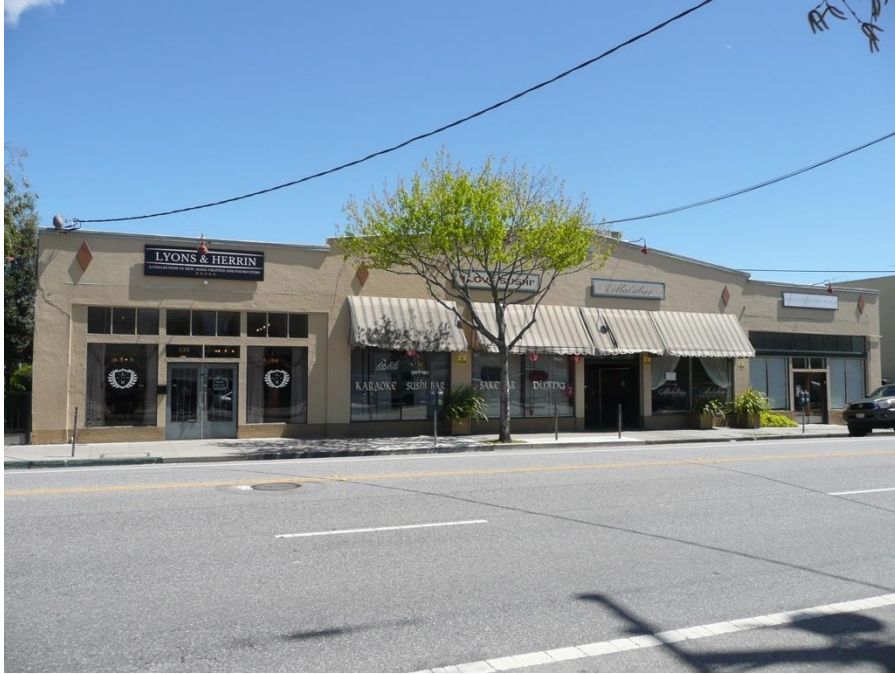
Figure 12: The west elevation of the 1926 building, facing east.
