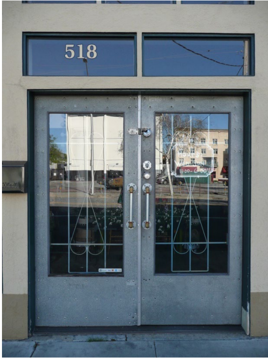
Detail of the contemporary metal double doors at the northernmost bay of the 1926 building.
