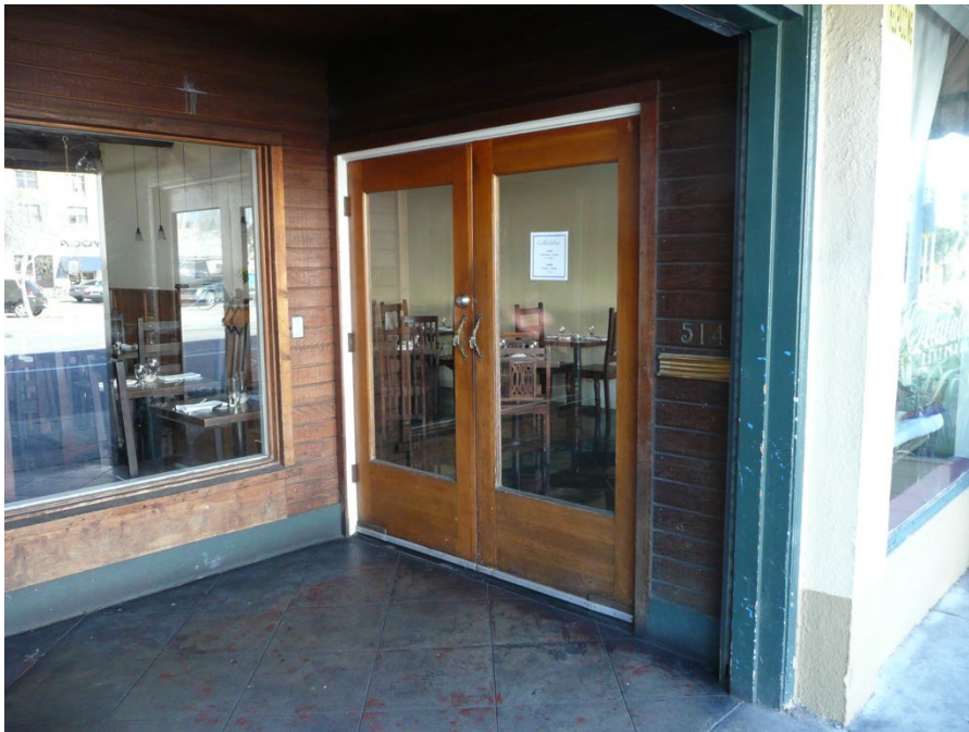
Detail of recessed opening within the center bay, showing the plate-glass window and north-facing double doors facing southeast.
