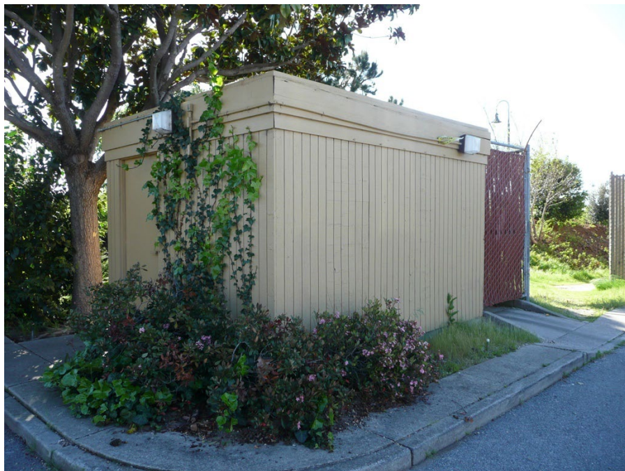
North and west elevations of the ca. 2007 Shed 2, facing southeast.
