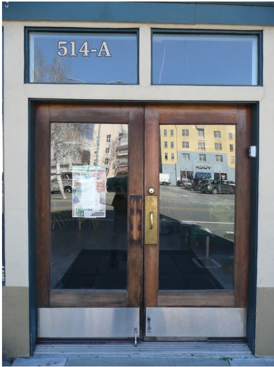
Detail of the contemporary doors and transom windows at the southernmost bay of the 1926 building.
