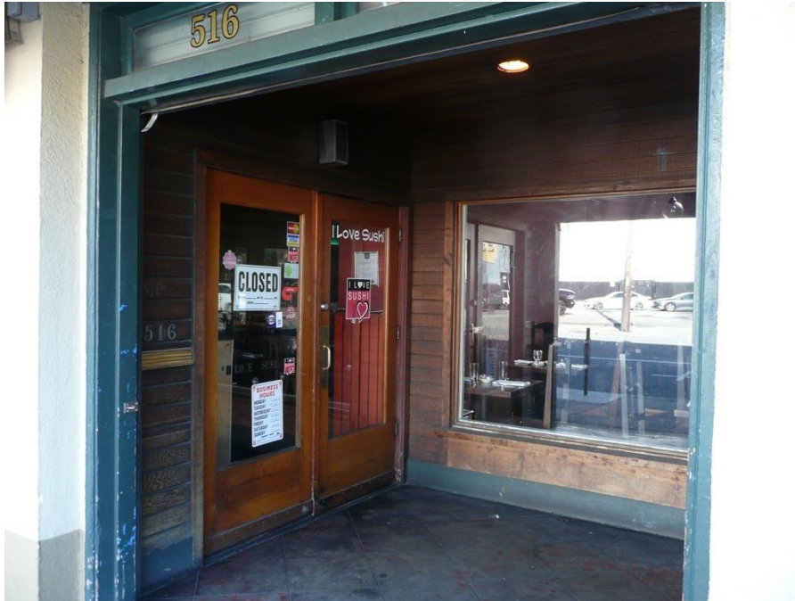
Figure 18: Detail of recessed opening within the center bay, showing the south-facing double doors and plate-glass window, facing northeast.
