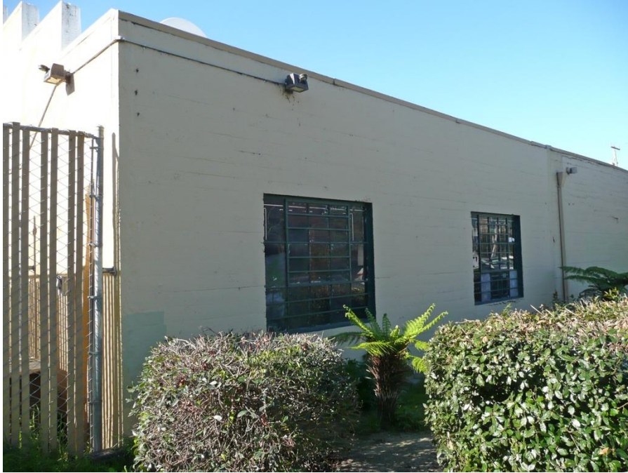
Figure 30: Detail of the two metal multi-light windows near the eastern end of the north elevation of the 1926 building, facing southwest.
