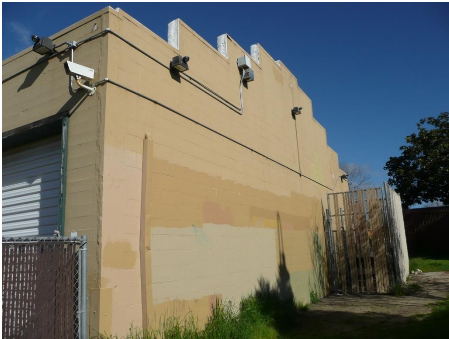
Figure 31: East elevation of the rear wing, facing north-northwest.
