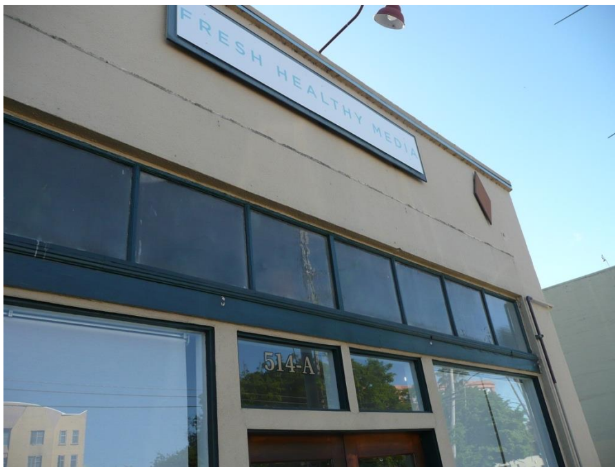
Figure 15: Detail of clerestory at the southernmost bay of the 1926 building, along the west elevation, facing southeast.
