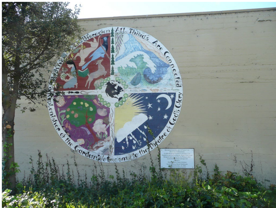
Detail of the contemporary painted mural at the north elevation of the 1926 building, facing south.
