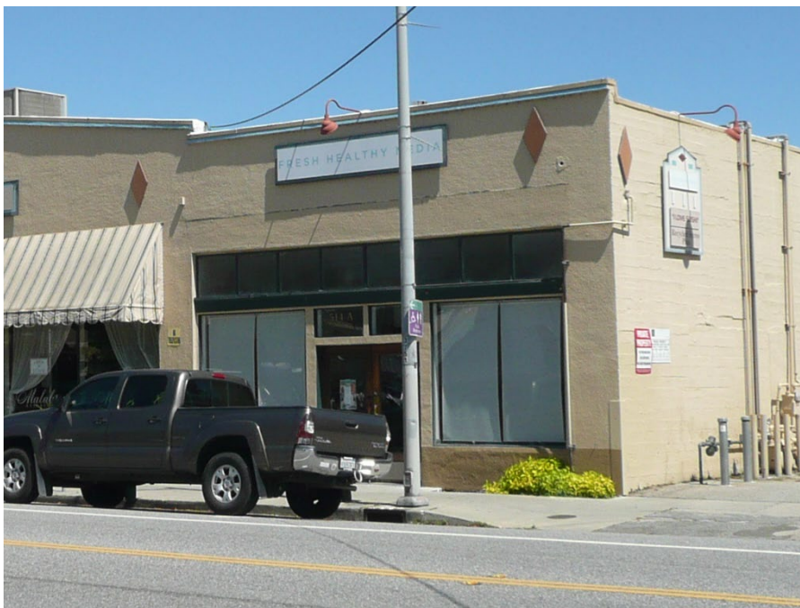
The west elevation at the southernmost bay, facing northeast.
