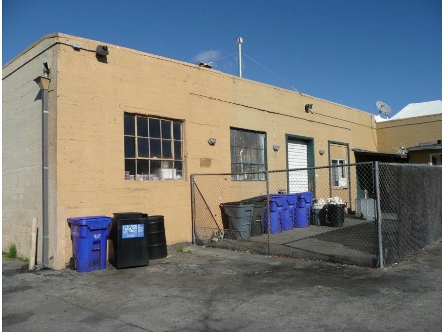
Figure 32: East elevation of the main building form, with the south elevation of the rear wing visible at far right, facing northwest.
