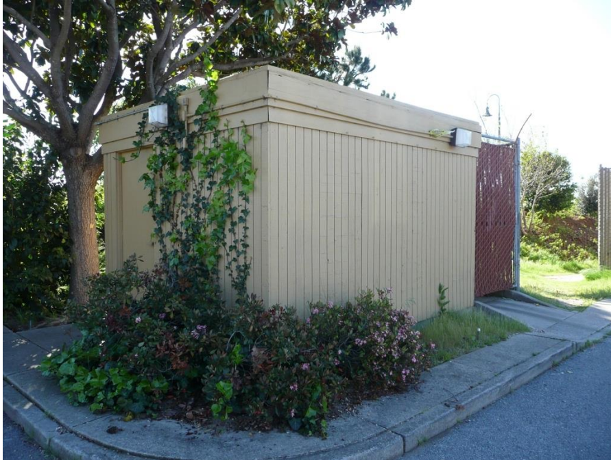
Figure 40: North and west elevations of the ca. 2007 Shed 2, facing southeast.
