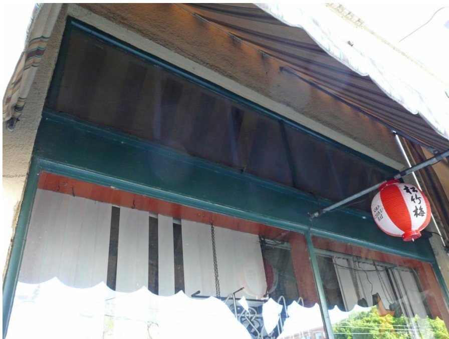
Figure 21: Detail of clerestory window above plate-glass storefront window at center bay of the 1926 building.
