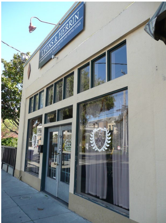
The northernmost bay at the west elevation of the 1926 building, facing north-northeast.
