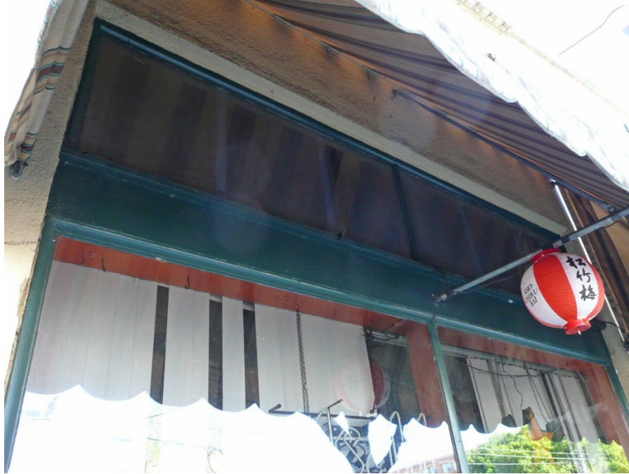
Detail of clerestory window above plate-glass storefront window at center bay of the 1926 building.
