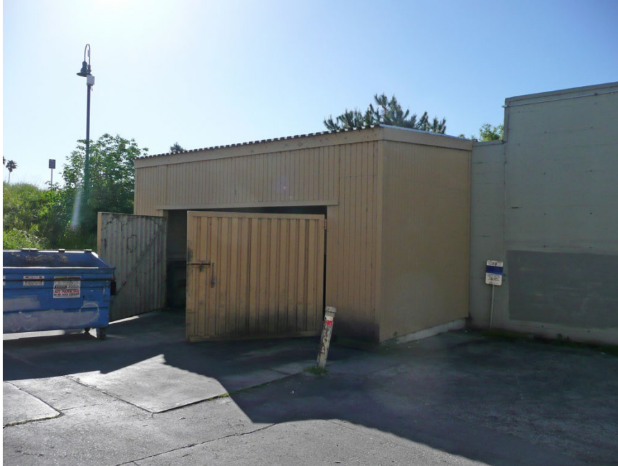
North and west elevations of the ca. 2007 Shed 1, with the neighboring building at 512 Front Street visible at right, facing southeast.
