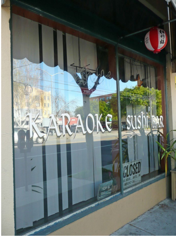
Detail of the pair of plate-glass windows located to the north of the recessed entry within the center bay of the 1926 building, facing southeast.
