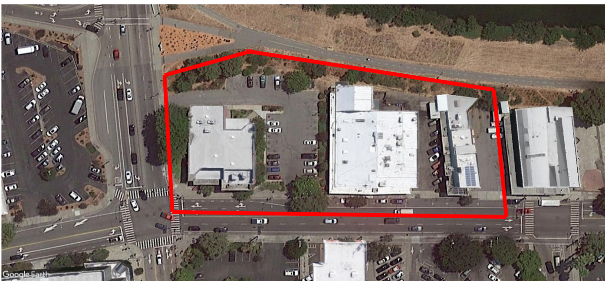
Image #1 - Proposed Mixed Use Project 530 Front Street – Approximate Project Boundaries (in red).
