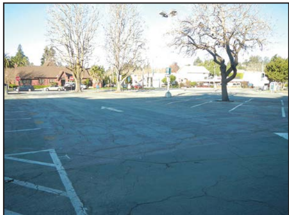
Photograph 6. Overview of the Parking lot, facing northwest.
