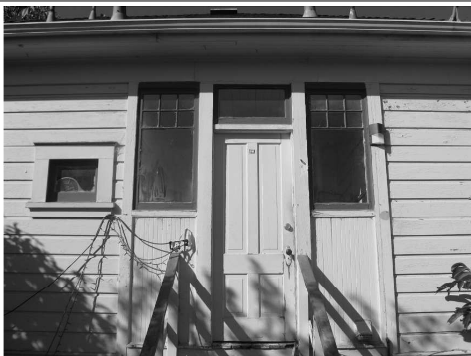
Photo 10: View of the rear entry.
