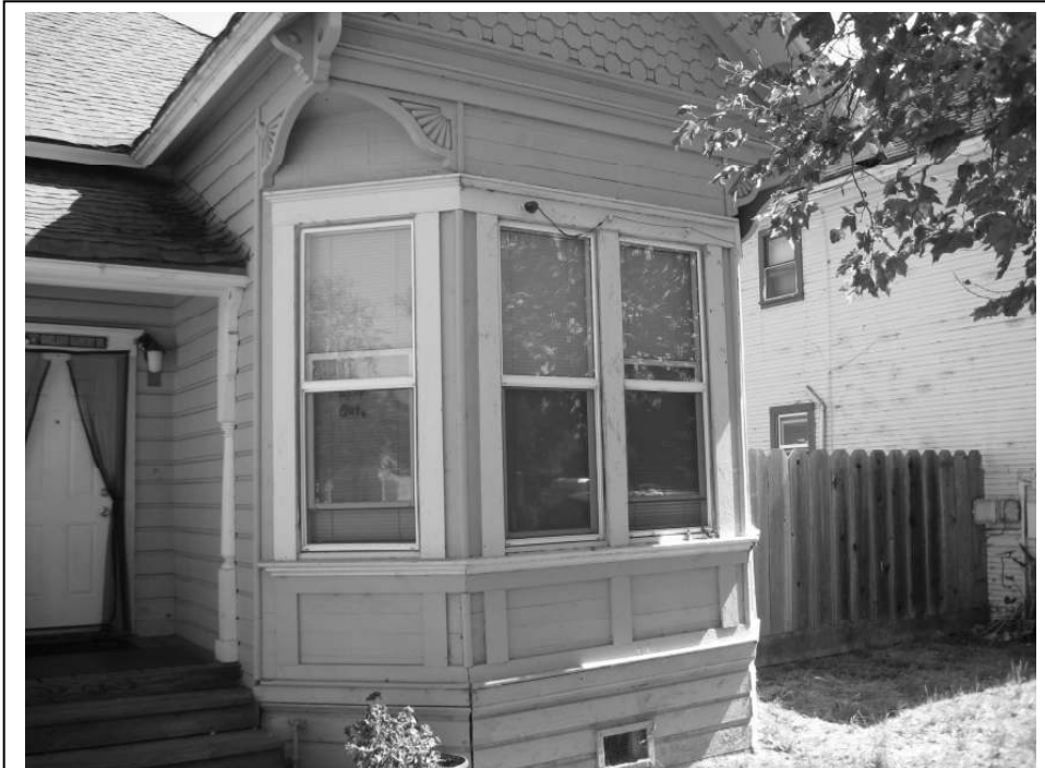
Photo 4: View of the large window bay on the front façade.
