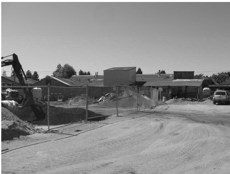
Photo 8: View of the rear façade.
