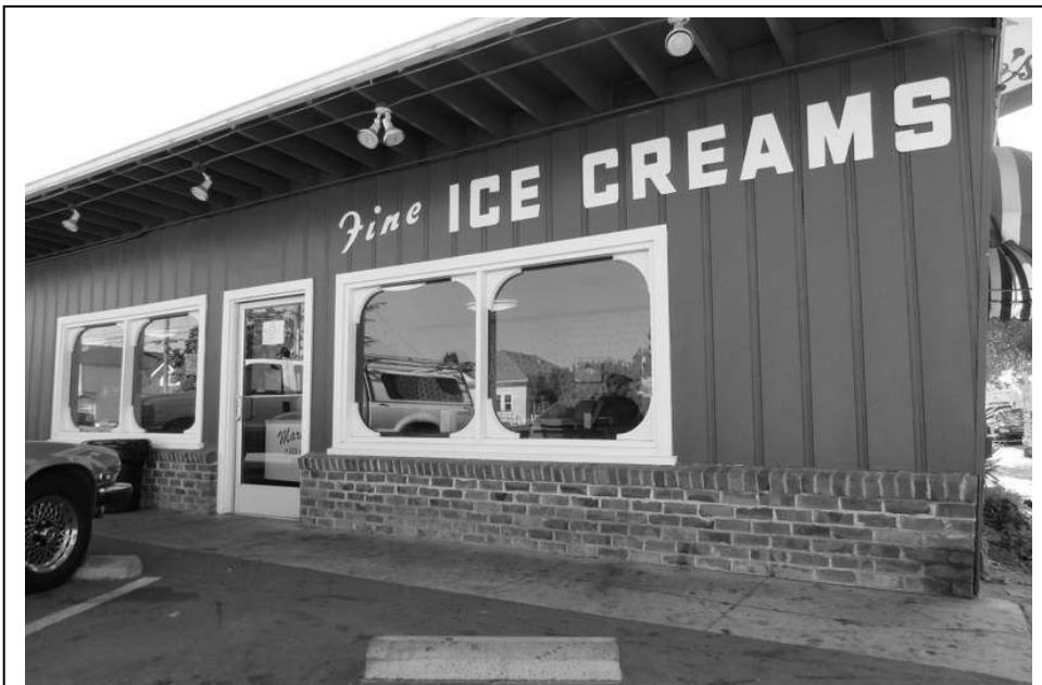
Photo 2: A closer view showing the main entrance.
