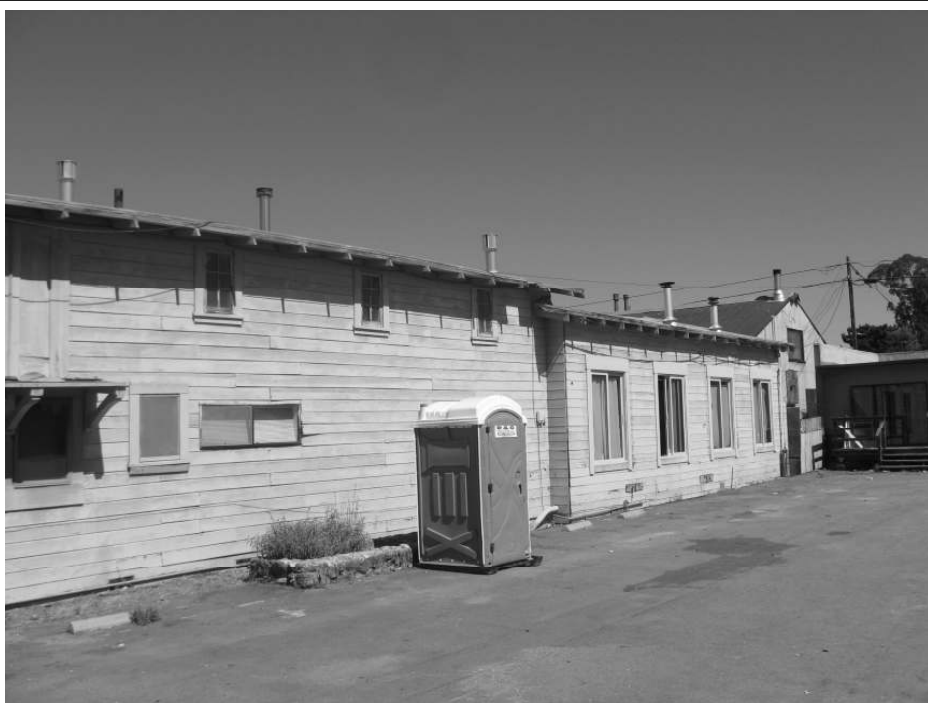
Photo 6: View along the southern façade.
