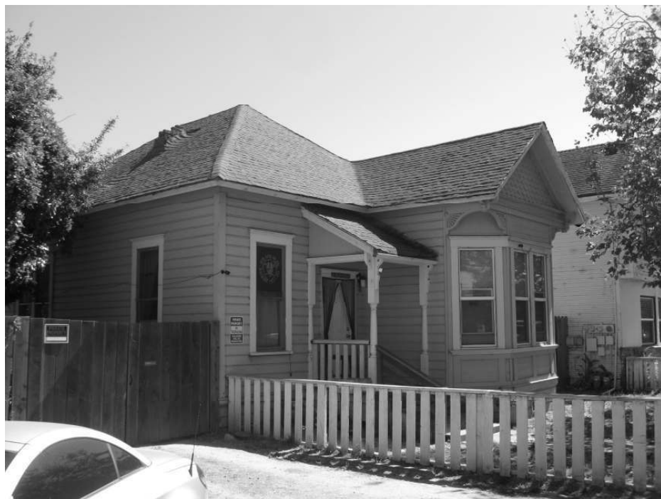
Photo 2: Oblique view of the front façade.
