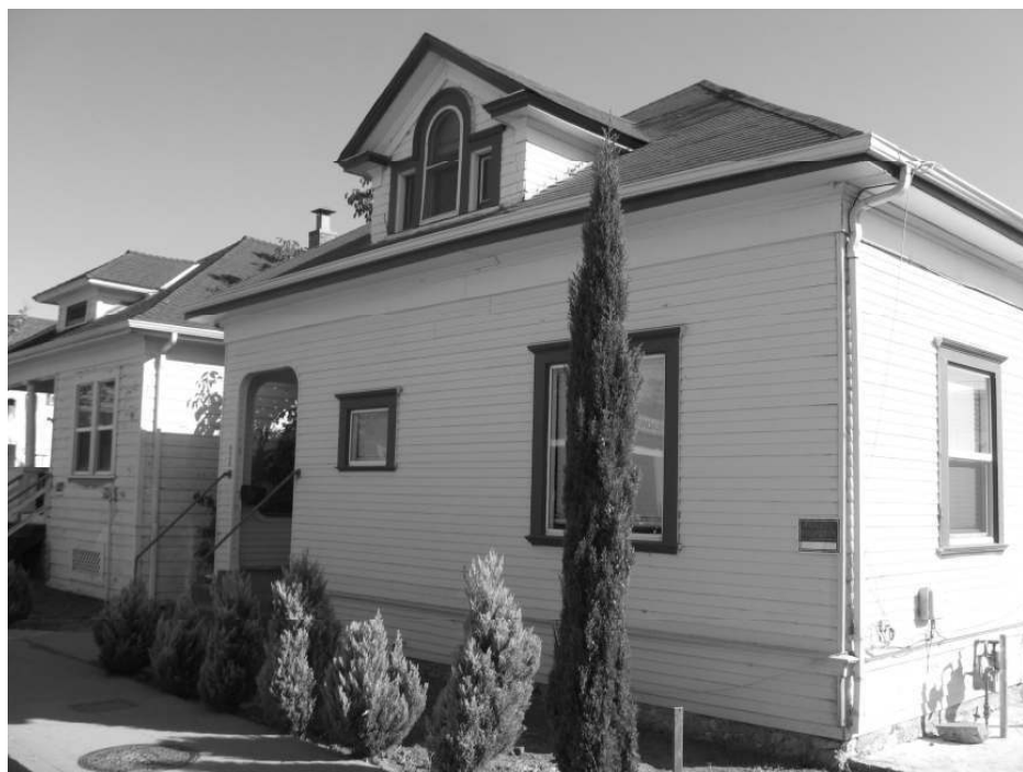
Photo 2: Another view of the front façade.
