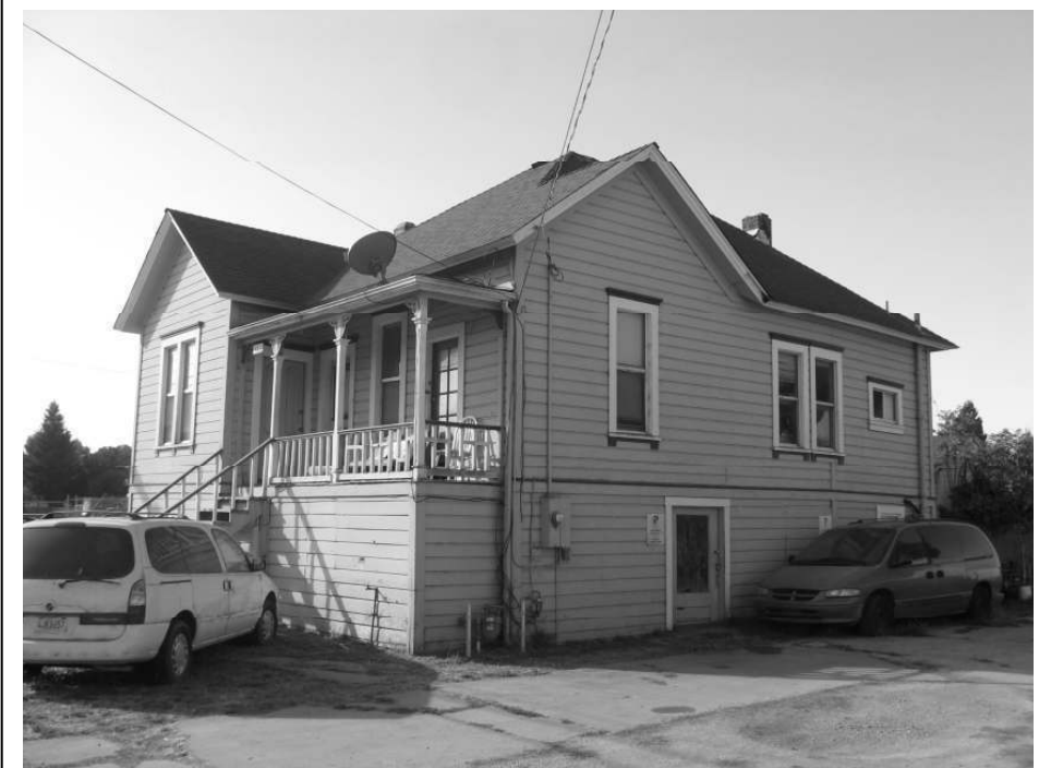
Photo 5: View of the northern façade of the residence.
