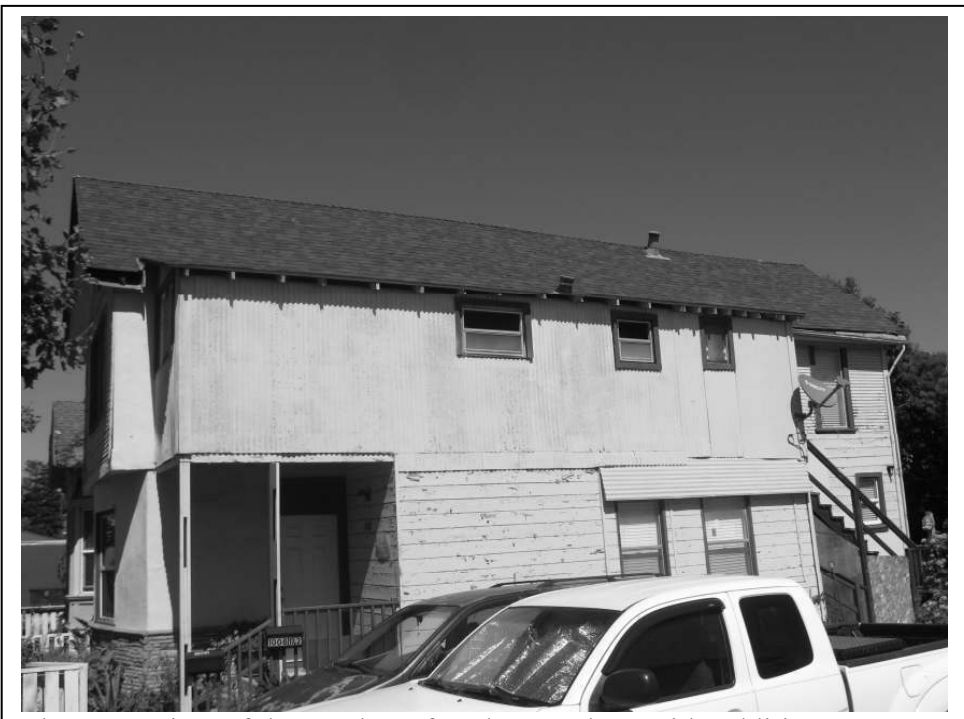
Photo 6: View of the southern façade, note large side addition.
