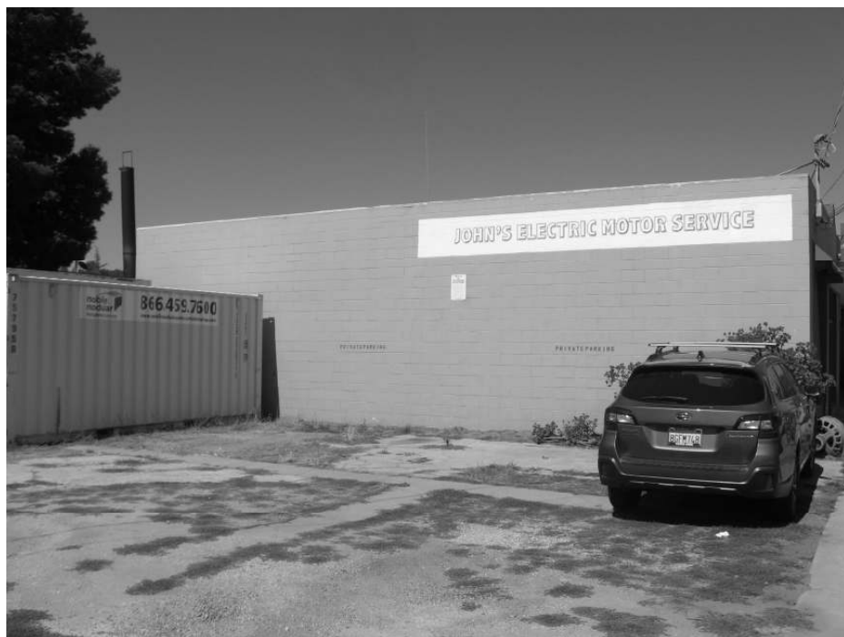
Photo 6: View of the southern façade.
