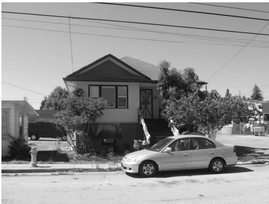
Photo 2: Another view of the front façade.
