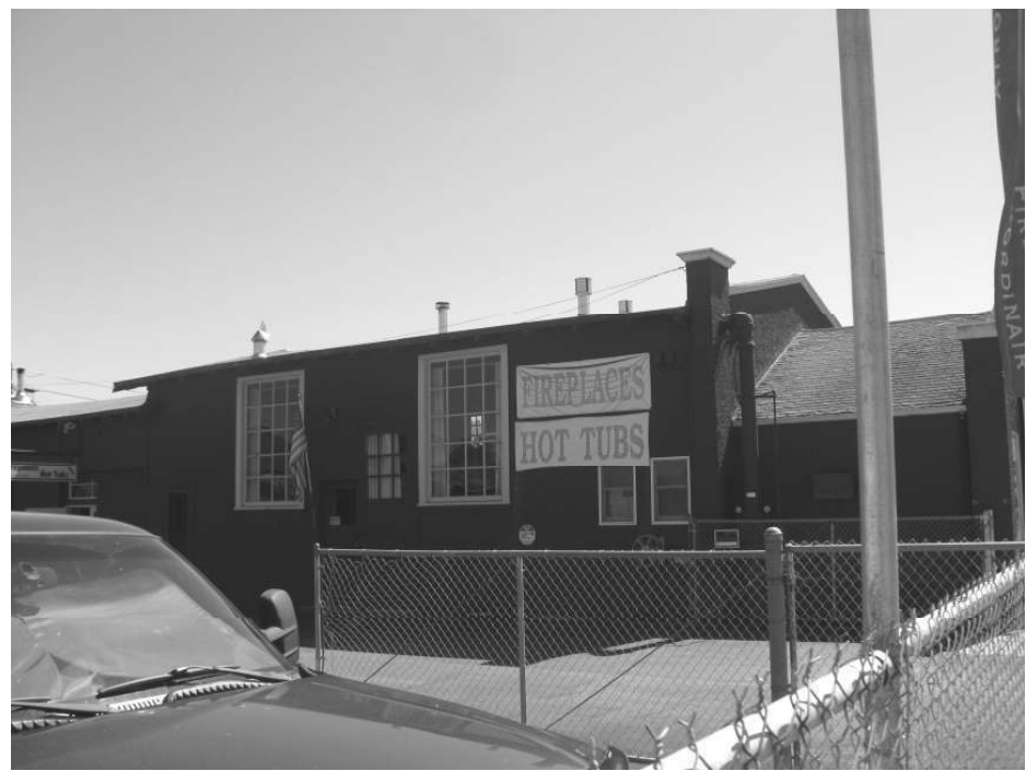
Photo 7: View of the northern façade of the sales area.
