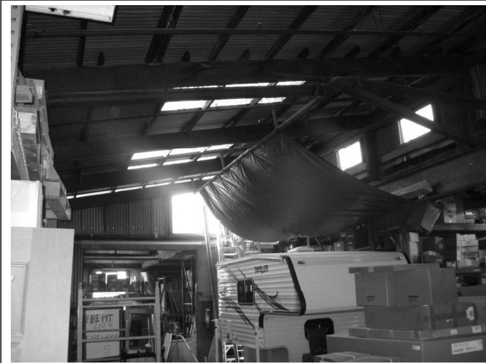
Photo 15: Another view of the warehouse area.
