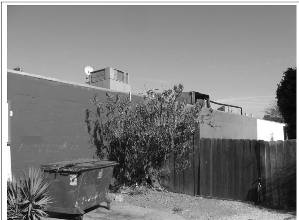
Photo 8: View of the rear portion of the southern façade.
