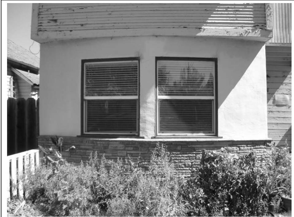
Photo 3: View of the lower story and window bay.
