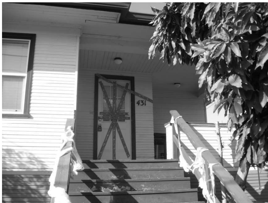
Photo 4: View of the entry and porch.
