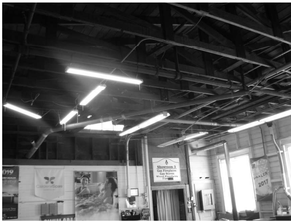
Photo 11: Interior view of the sales office showing rafter trusses.
