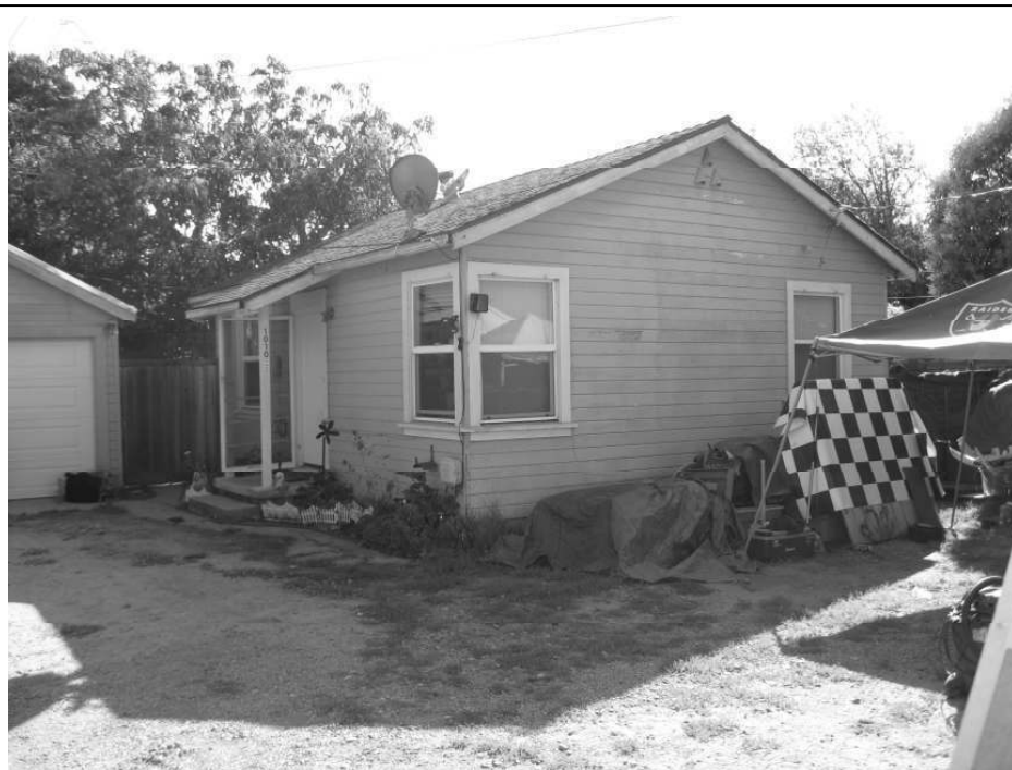
Photo 10: View of the small secondary unit on the property (post 1950).
