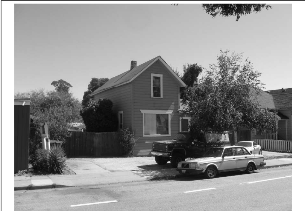
Photo 1: View of the front façade of 1014 Ocean Street from the northwest.
