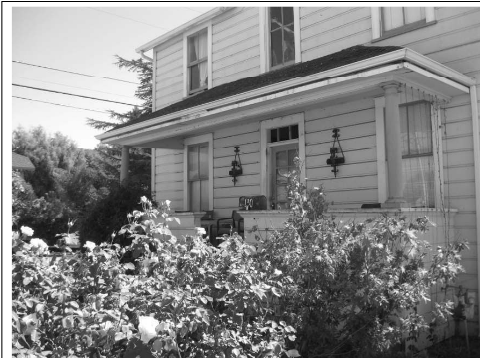
Photo 2: View of the front porch and entry.
