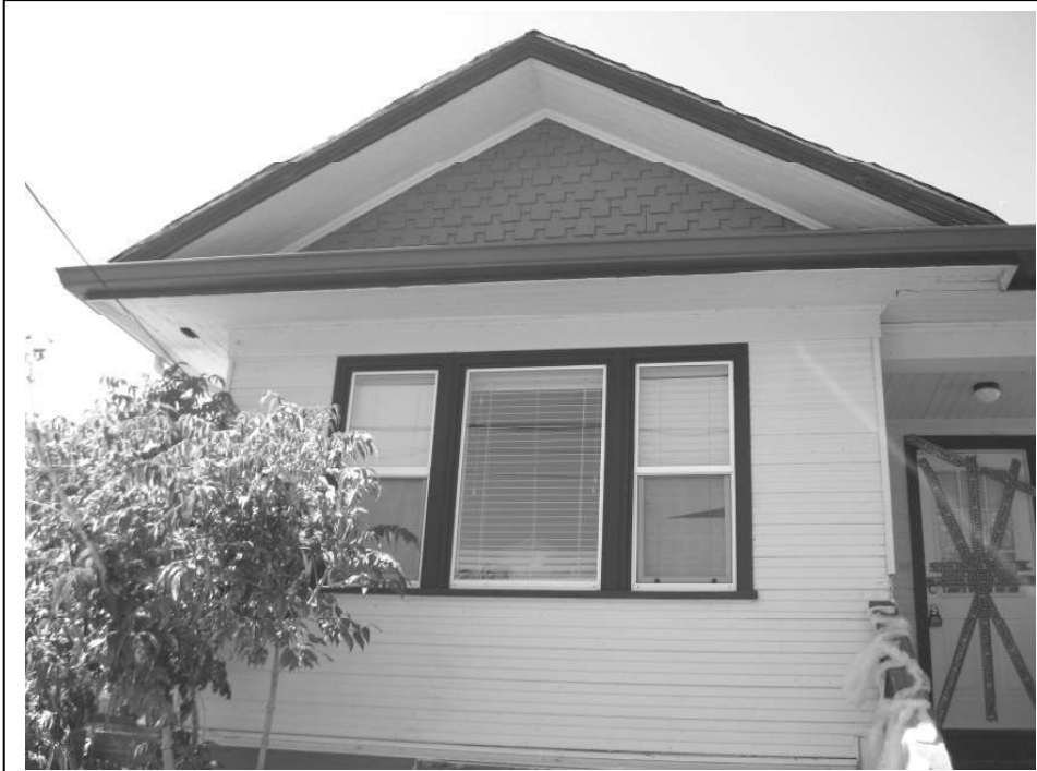
Photo 3: View of the front gabled (southern) wing.
