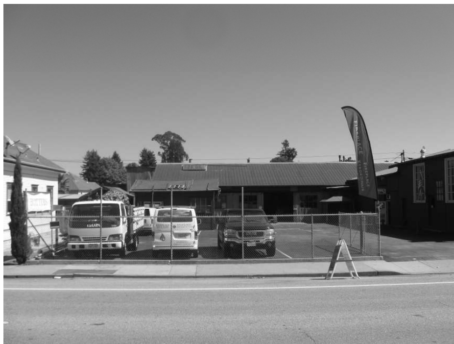
Photo 4: View of the northern wing from Ocean Street.
