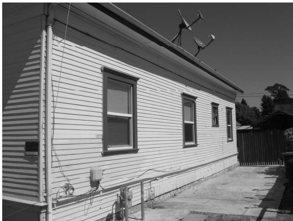
Photo 4: View along the southern façade.
