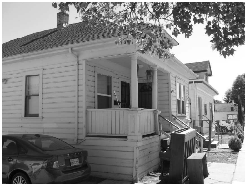
Photo 4: Oblique view showing the northwest corner of the structure.
