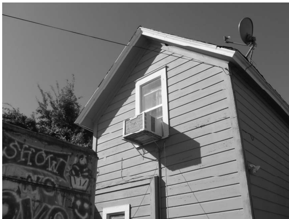
Photo 6: View of the rear façade of the residence.
