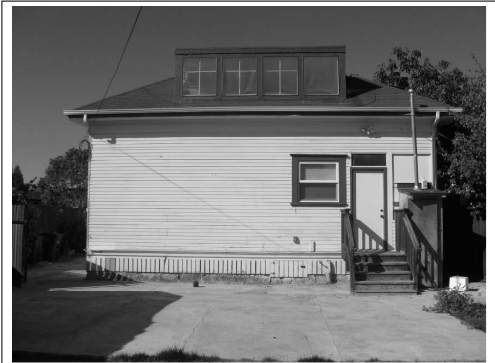
Photo 7: View of the rear façade.
