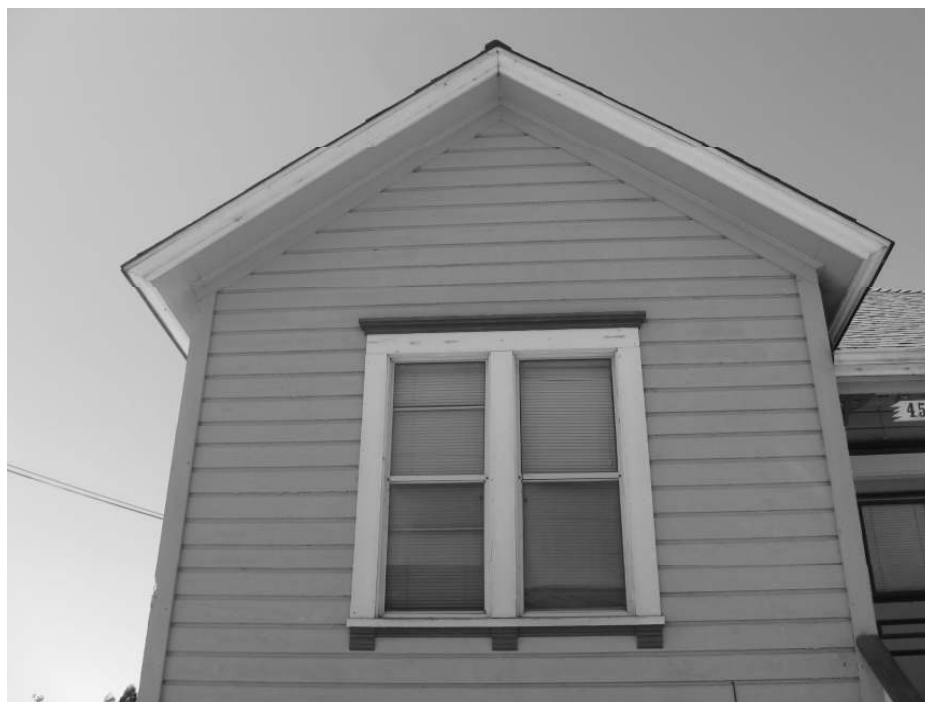
Photo 4: View of the front gabled (southern) wing.
