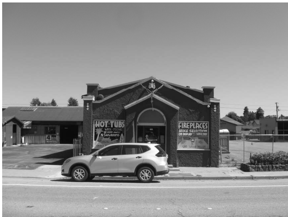
Photo 2: View of the store front of the structure.
