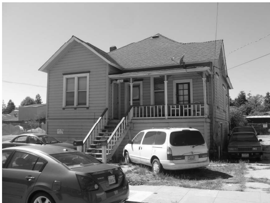
Photo 2: Another view of the front façade.
