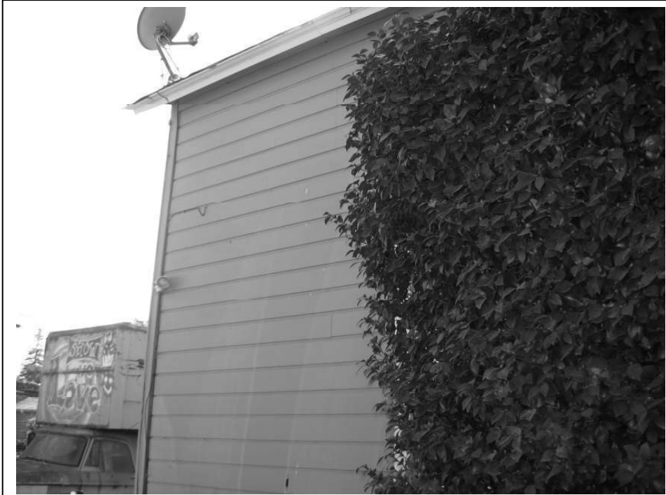
Photo 7: View of the rear portion of the northern façade.
