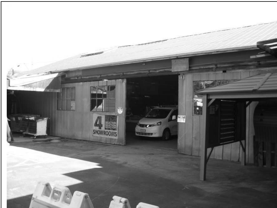
Photo 12: View of the entry to the warehouse area.
