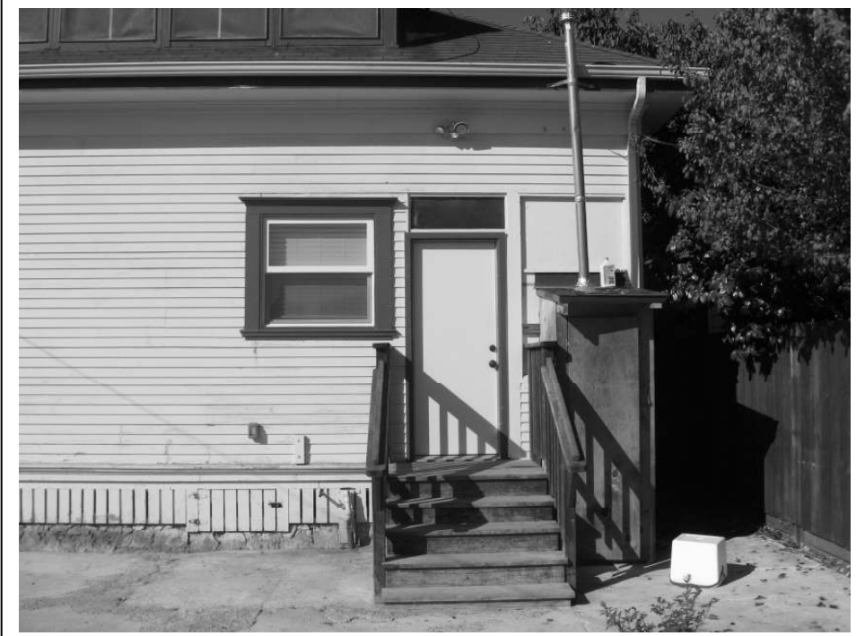
Photo 9: View of the rear entry.
