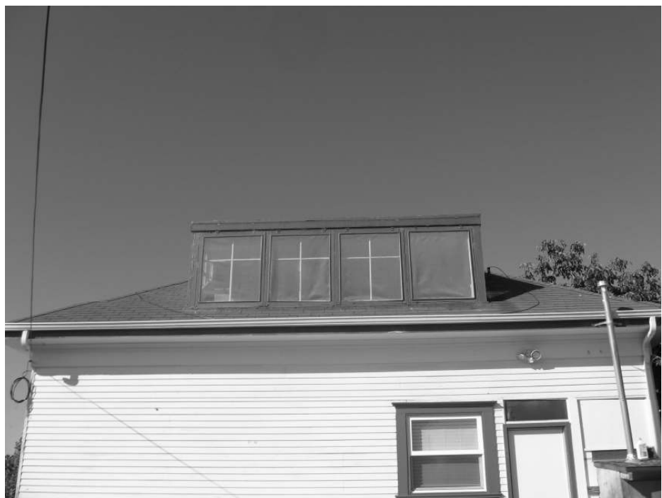
Photo 8: View of large rear informal dormer.
