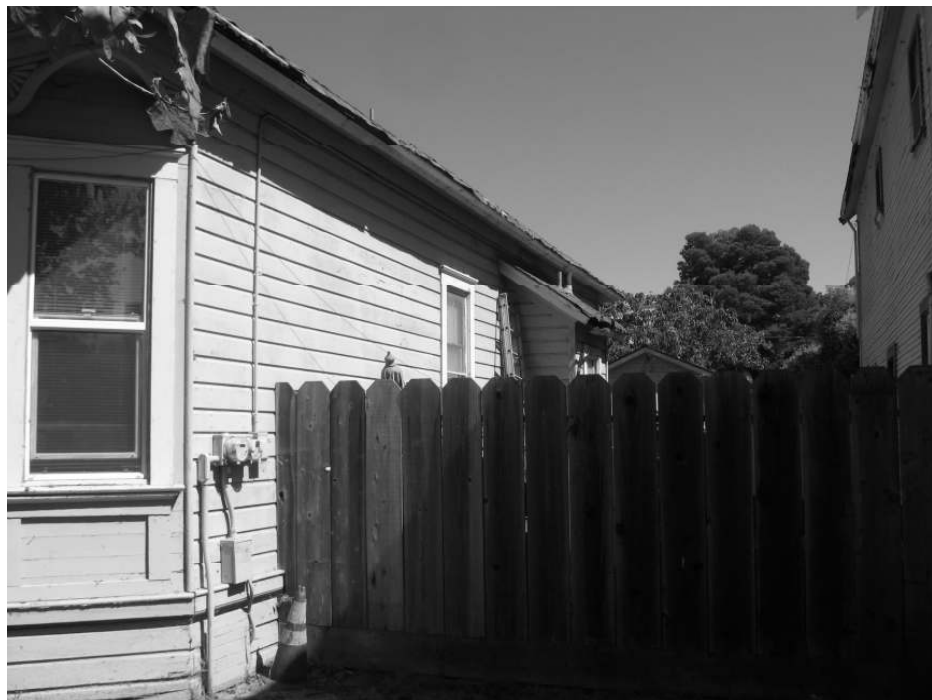
Photo 6: View along the southern façade of the residence.
