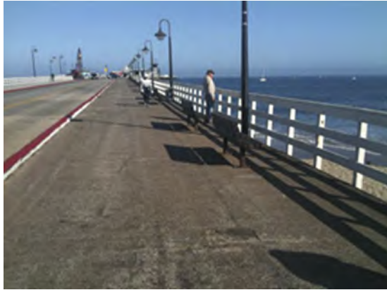
West Walkway Near Entrance
