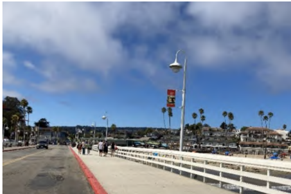
East Walkway Looking Toward Wharf Entrance
