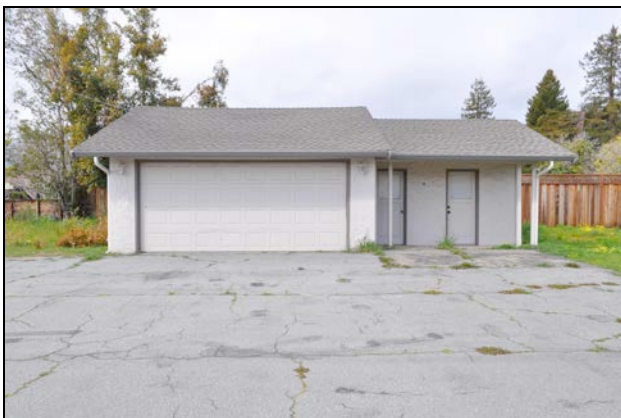
Figure 5. South elevation of detached garage.
