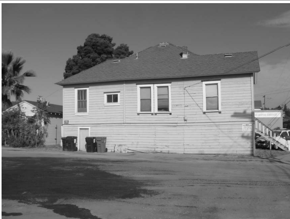
Photo 6: View of the southern façade.
