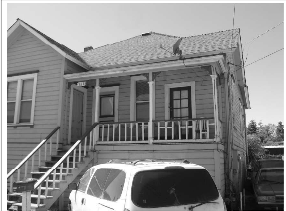
Photo 3: View of the front porch and entry.
