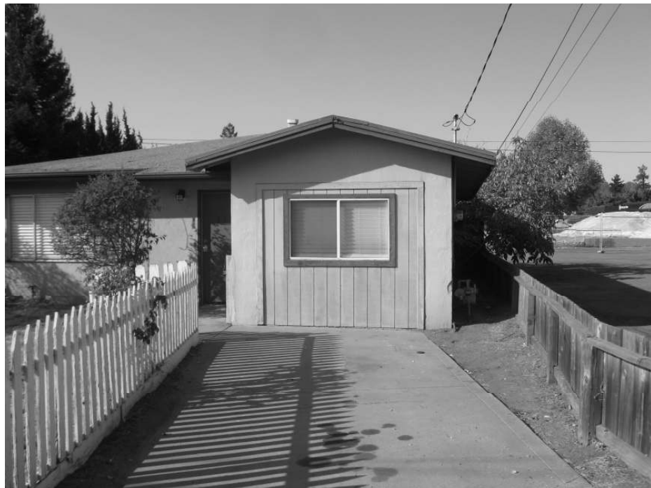
Photo 2: View of the extending front gabled wing (converted garage).
