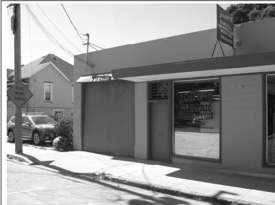
Photo 3: View of the garage bay and southern portion of the façade.
