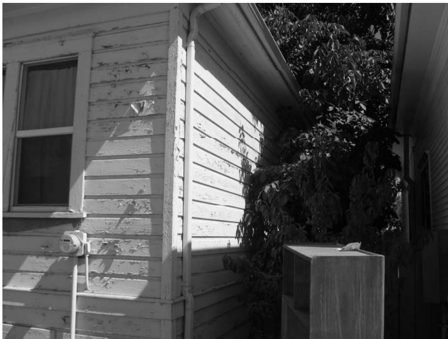
Photo 8: View of the (mostly obscured) southern façade.
