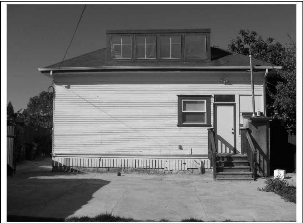
Photo 7: View of the rear façade.
