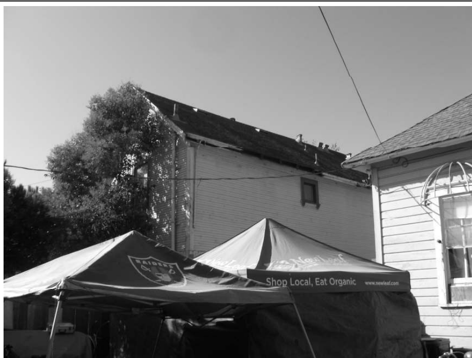
Photo 10: View of the rear portion of the home from the northeast.
