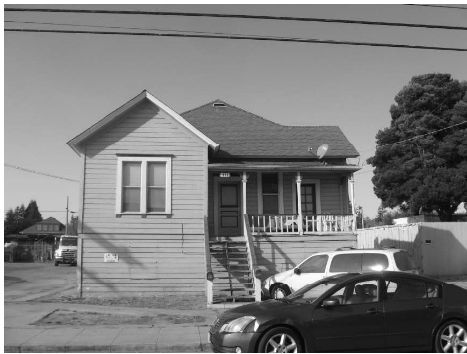
Photo 1: View of the front façade of 451 May Avenue
