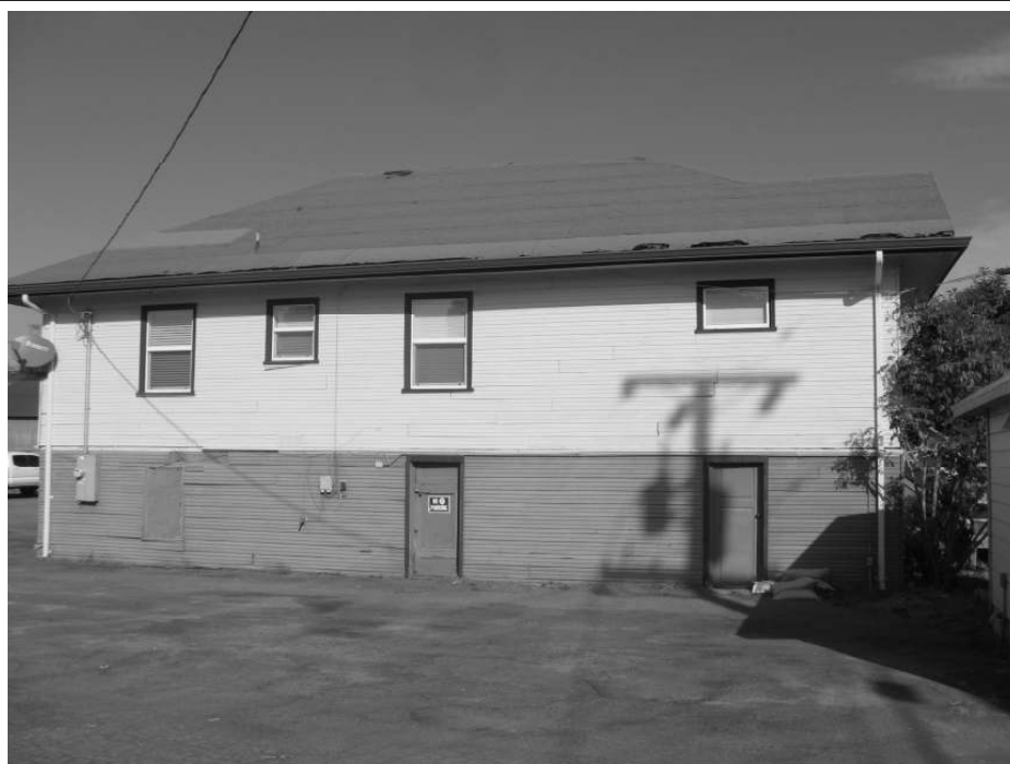
Photo 6: View of the southern façade of the residence.
