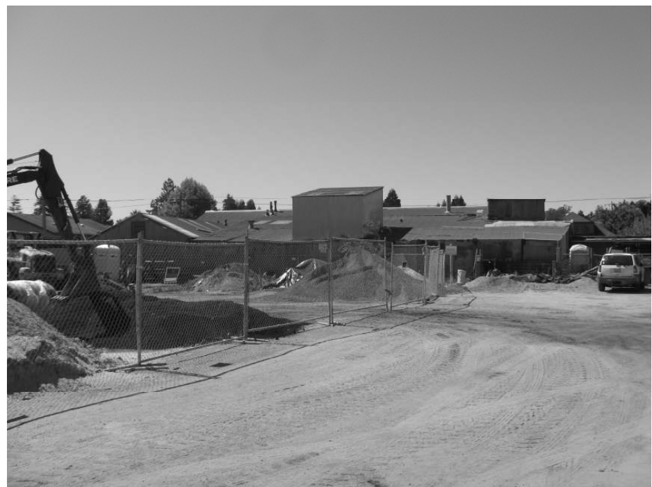
Photo 8: View of the rear façade.
