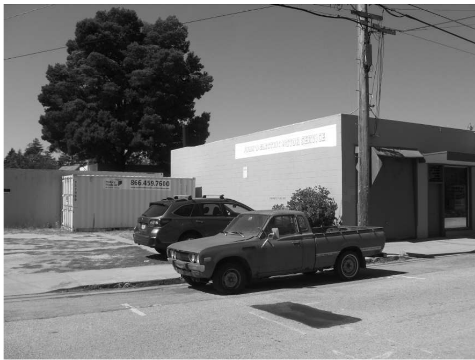
Photo 5: Oblique view of the southeast corner of the structure.
