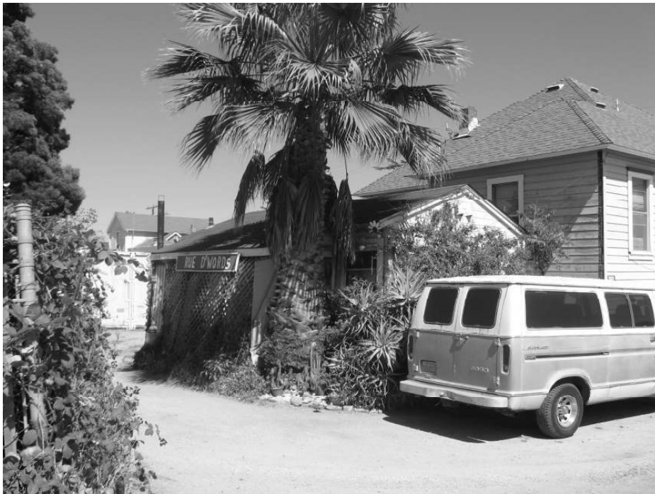
Photo 8: View of the secondary unit and rear façade of the main residence..
