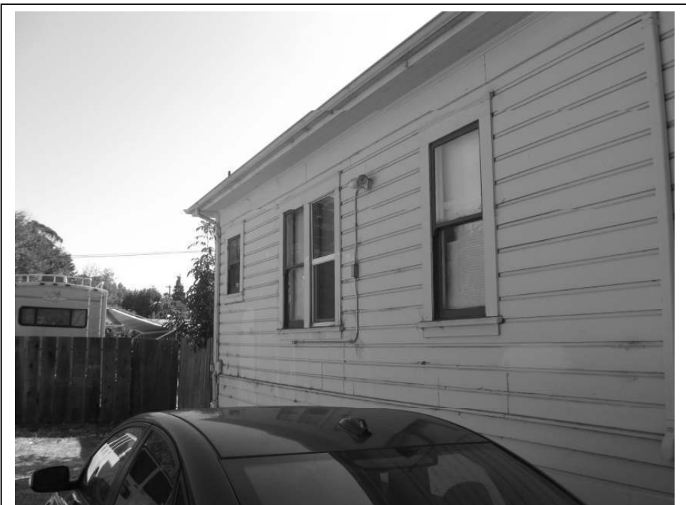
Photo 6: View of the rear portion of the northern façade.
