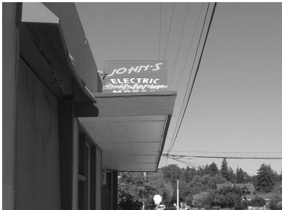
Photo 8: Detail of the cantilevered awning and sign.
