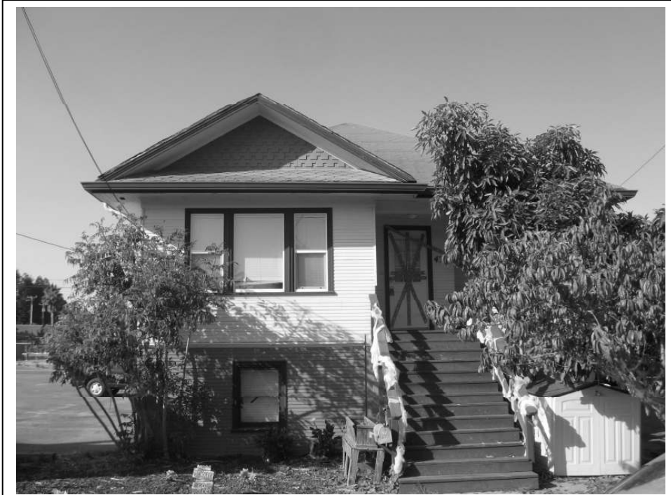
Photo 1: View of the front façade of 431 May Avenue
