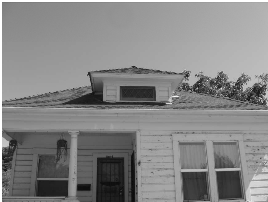
Photo 2: View of the centrally placed dormer.
