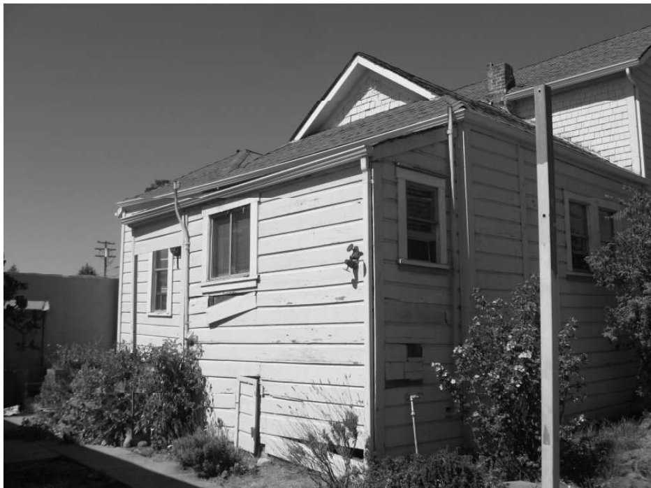
Photo 6: View of the rear façade showing later rear addition.
