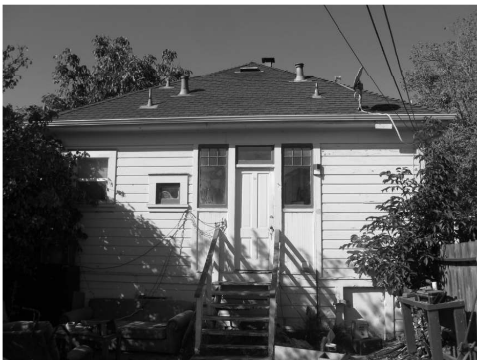
Photo 9: View of the rear of the structure.
