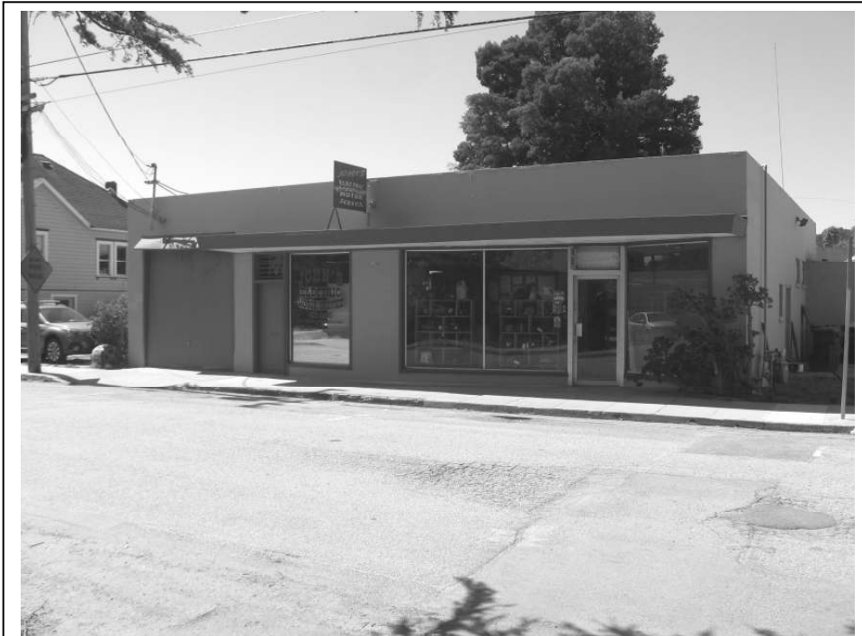
Photo 1: View of the front façade of 457 May Avenue
