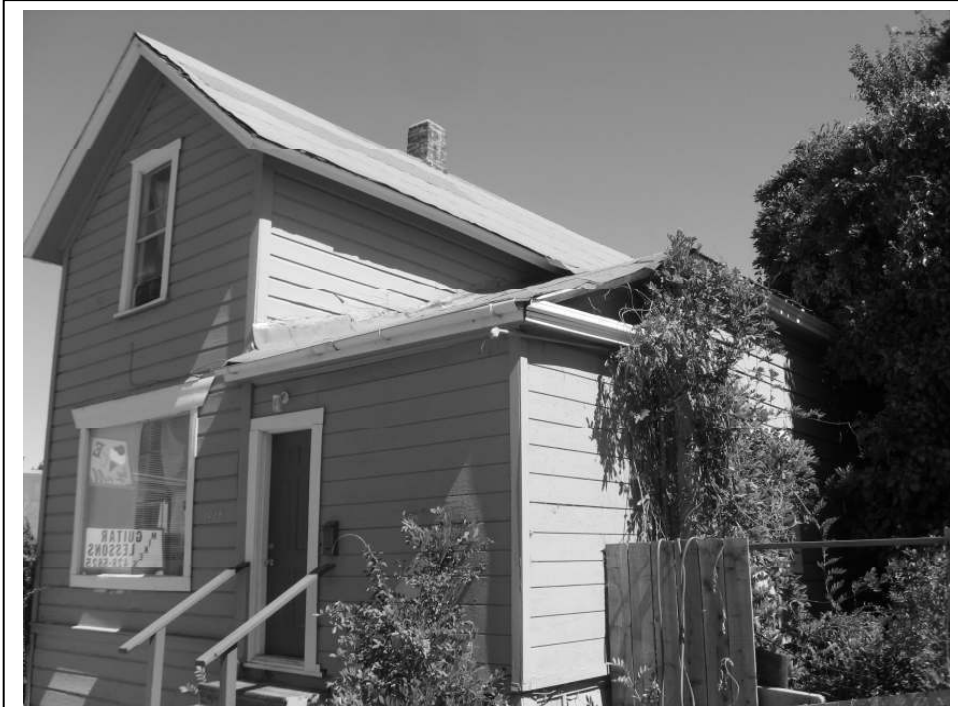
Photo 5: Oblique view of the residence from the southwest.
