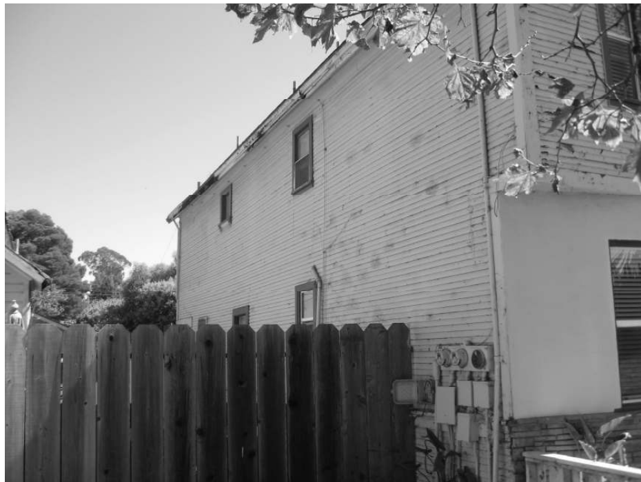
Photo 5: View along the northern façade.
