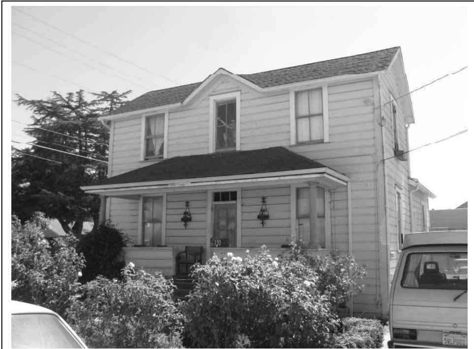
Photo 1: View of the front façade of 130 Hubbard Street
