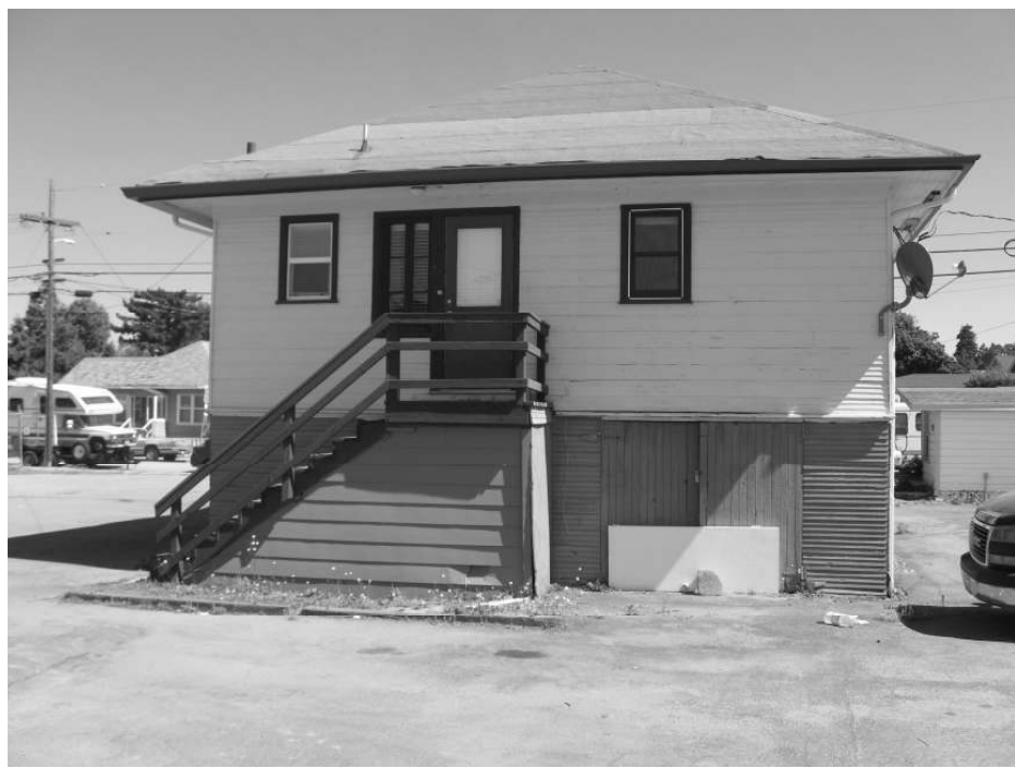
Photo 7: View of the rear façade and rear entry.
