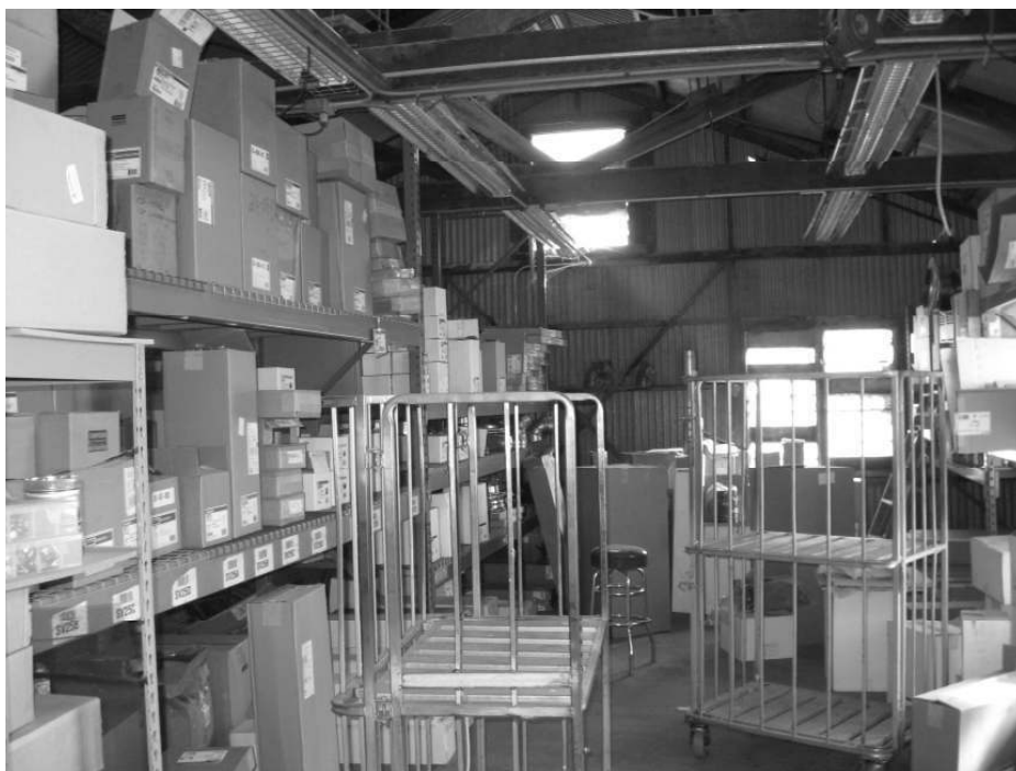
Photo 16: View of the warehouse area showing rafter trusses.
