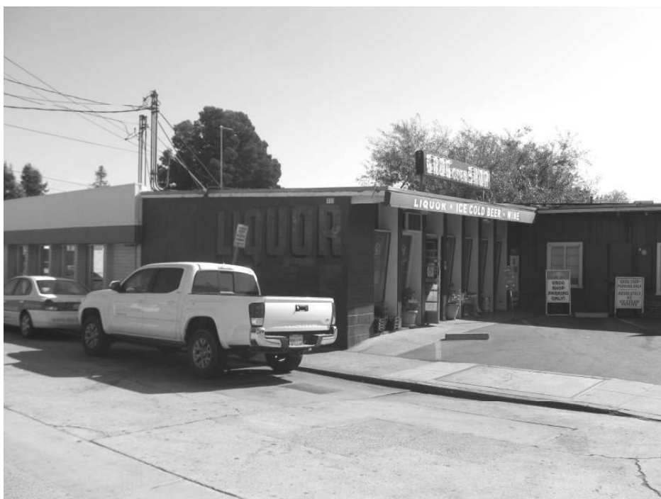
Photo 9: View of The Grog Shop addition.
