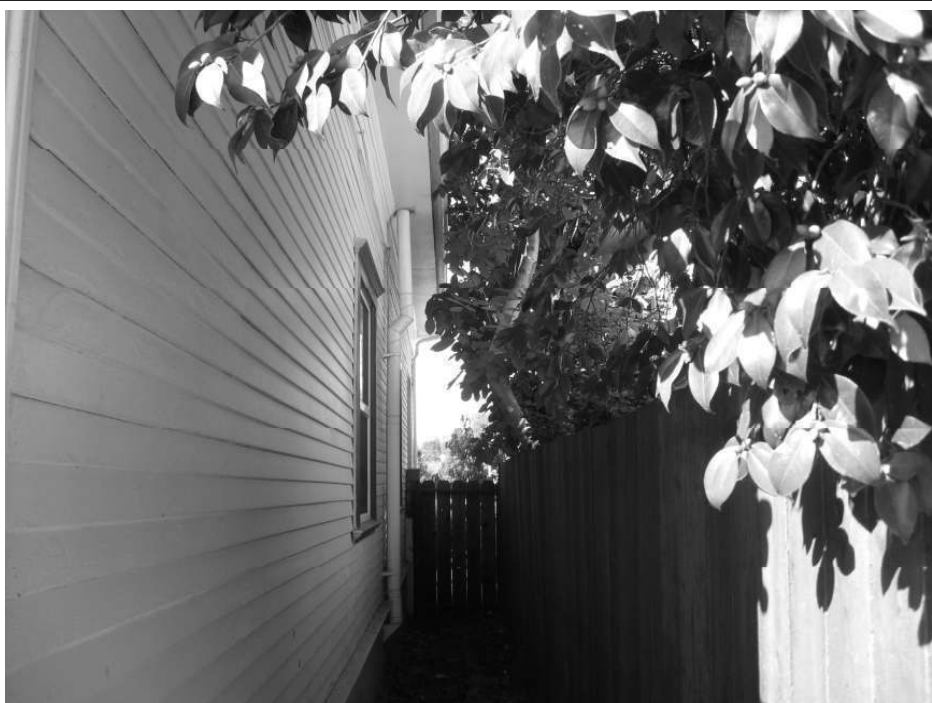
Photo 6: View along the northern façade from the rear.
