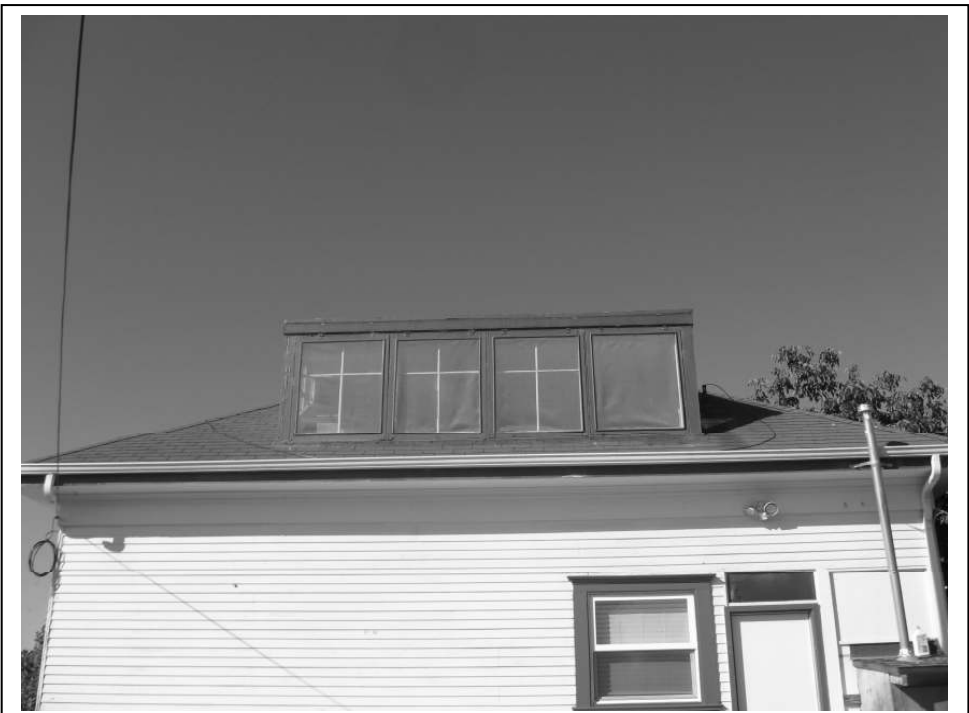
Photo 8: View of large rear informal dormer.
