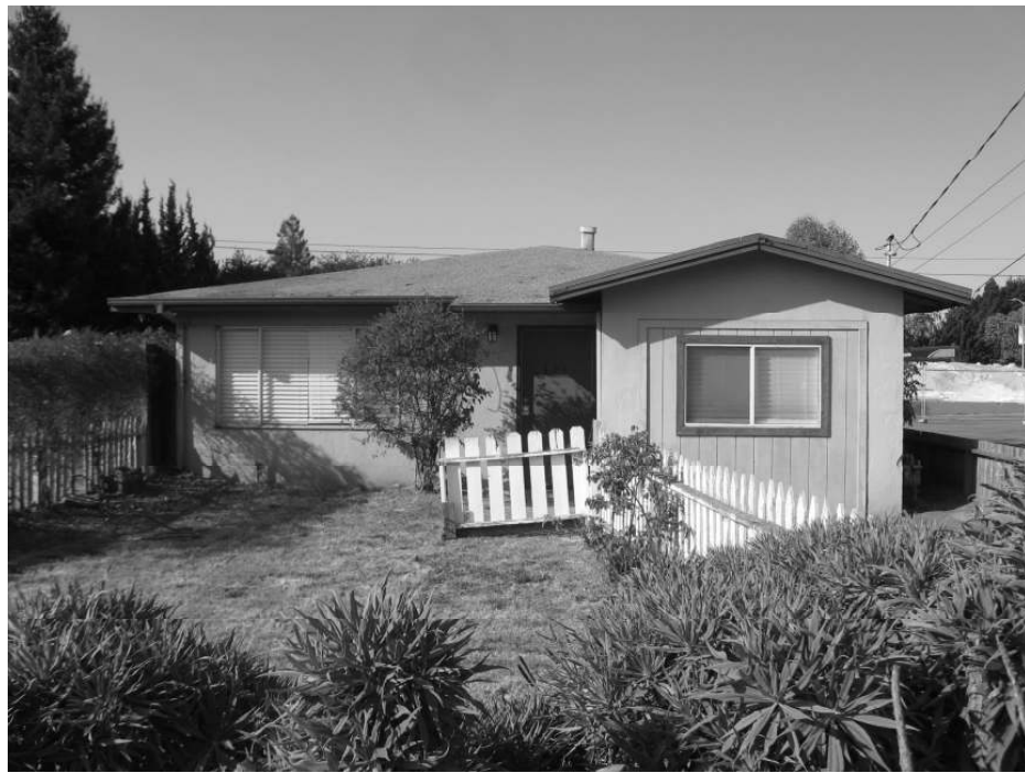
Photo 1: View of the front façade of 423 May Avenue
