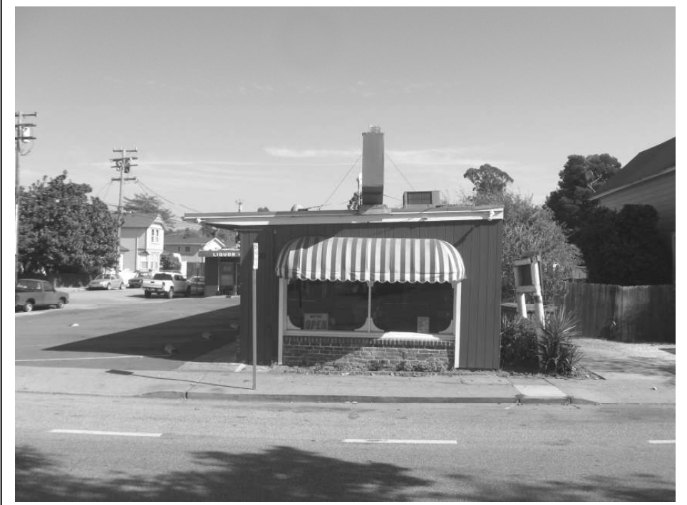
Photo 5: View of the western façade from Ocean Street.
