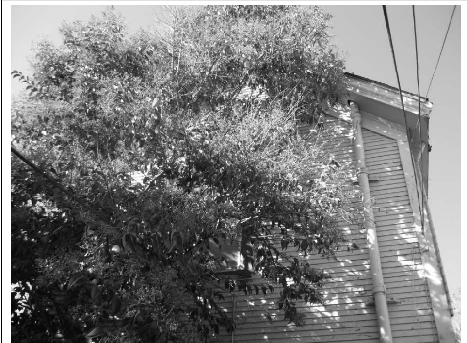
Photo 11: View of the upper portion of the rear of the residence.
