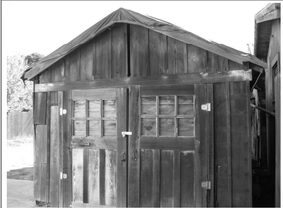
Photo 11: View of the front façade of the shed/garage.
