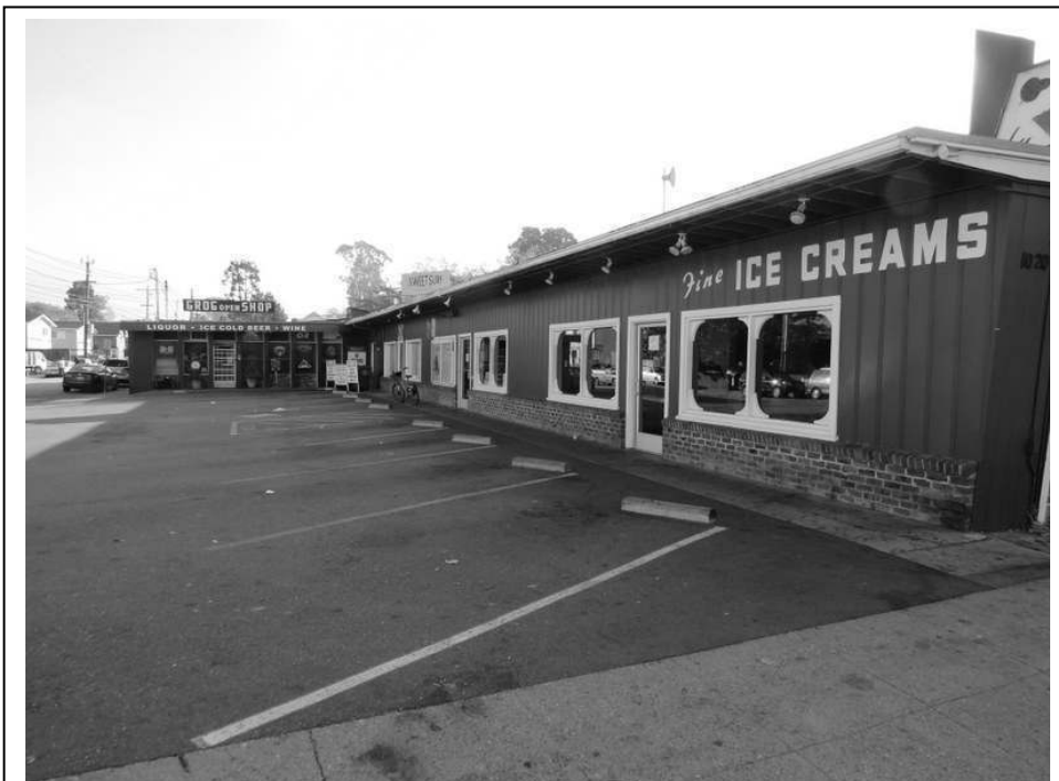
Photo 4: View along the original portion of the structure.
