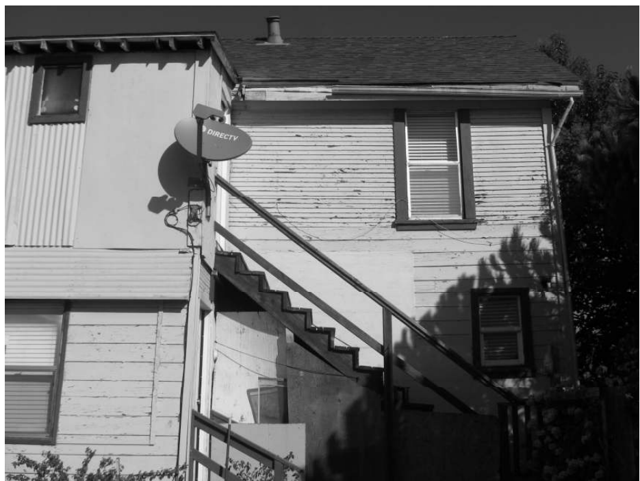
Photo 8: View of the rear entries on the southern façade.
