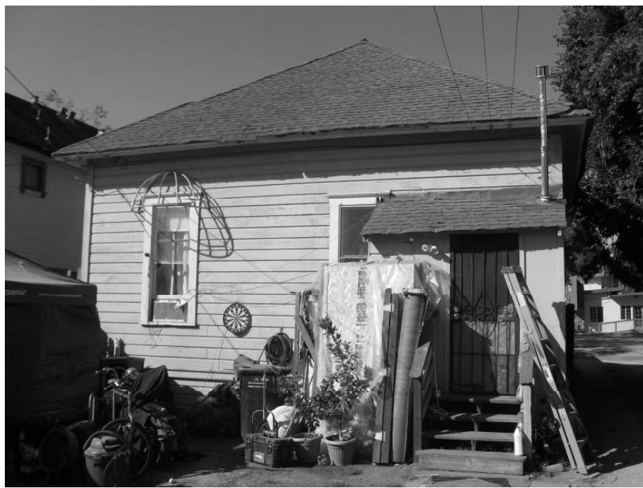
Photo 9: View of the rear of the residence, note small rear entry addition.
