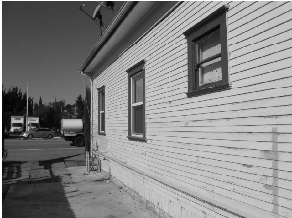
Photo 5: View along the southern façade from the rear.
