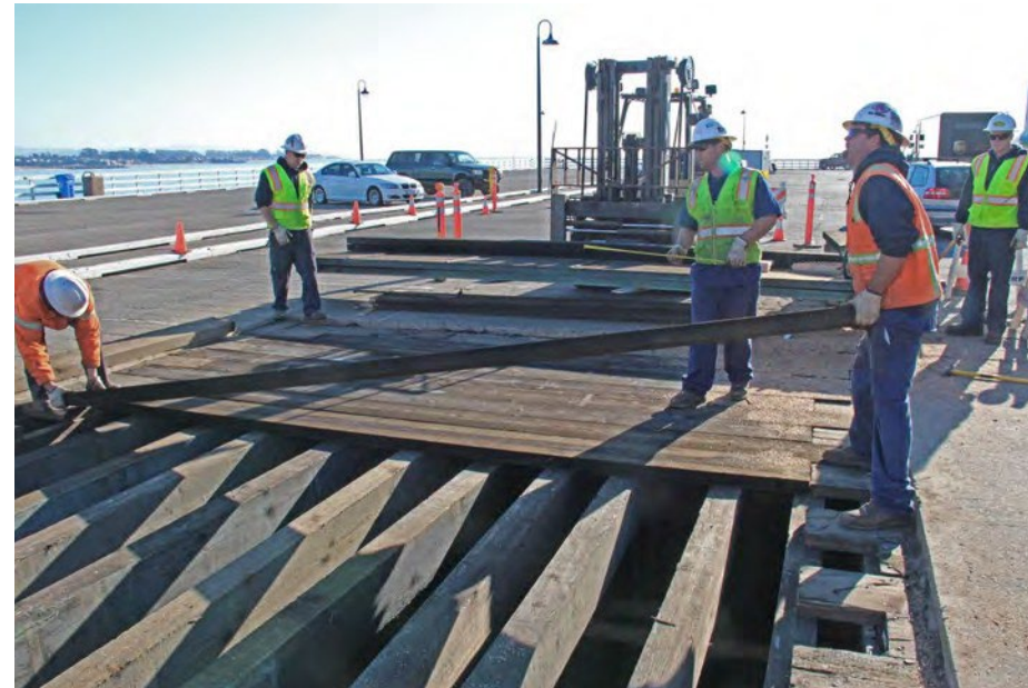
The Wharf is one of the longest pile-supported timber structures in the world and due to the on-going maintenance by Wharf staff it continues to be in serviceable and sound condition.
