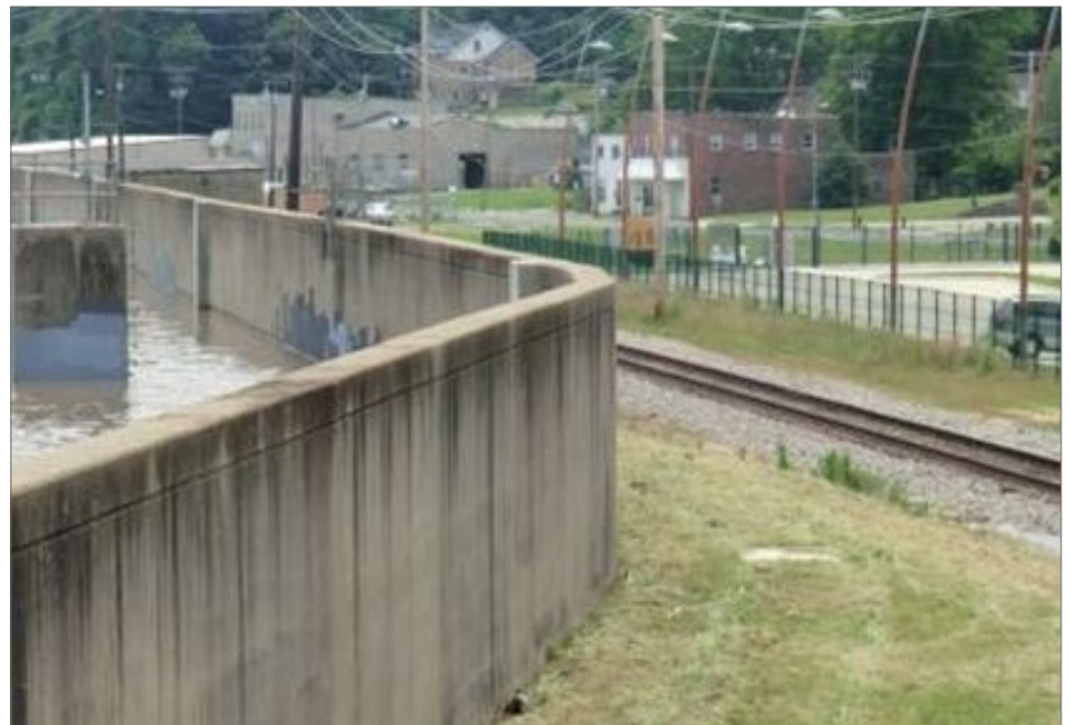
CONCRETE FLOODWALL, CAPE GIRARDEAU FLOOD PROTECTION PROJECT, CAPE GIRARDEAU, MISSOURI.
