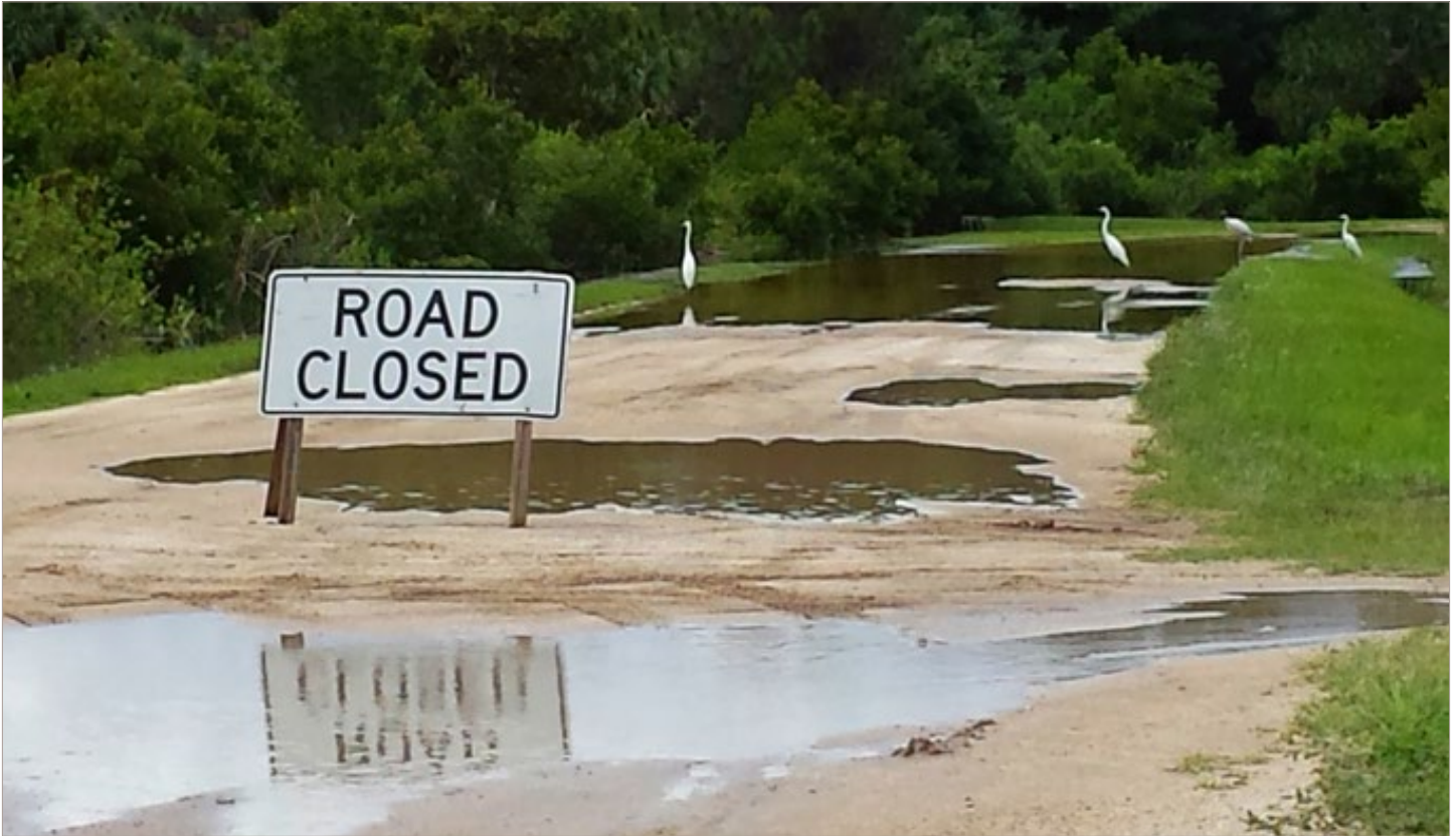
A FLOODED ROADWAY (SOURCE: ISTOCK).
