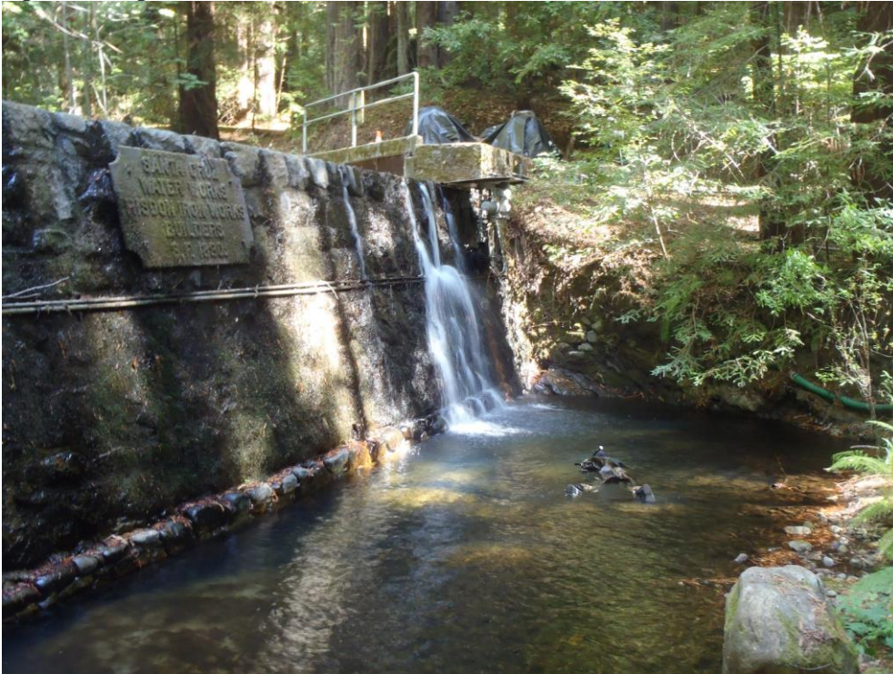
Photo: Laguna Creek Diversion from right bank downstream looking across the channel
