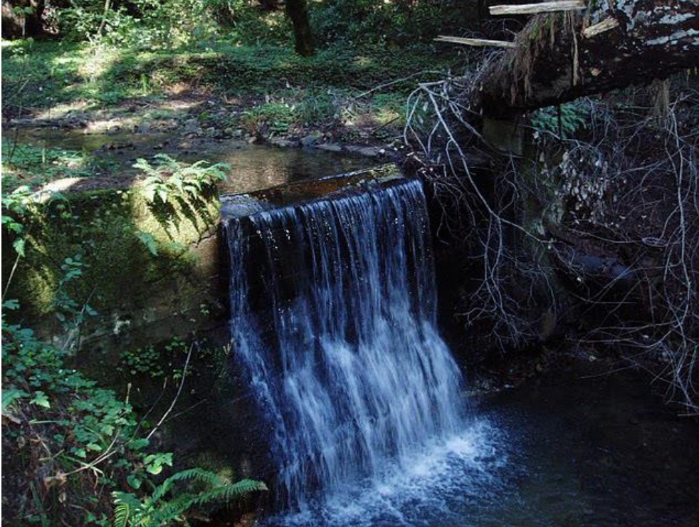
Photo: Reggiardo Diversion from right bank downstream looking across the channel
