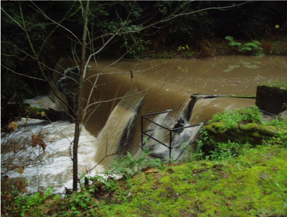
Photo: Majors Diversion from left bank downstream looking across the channel
