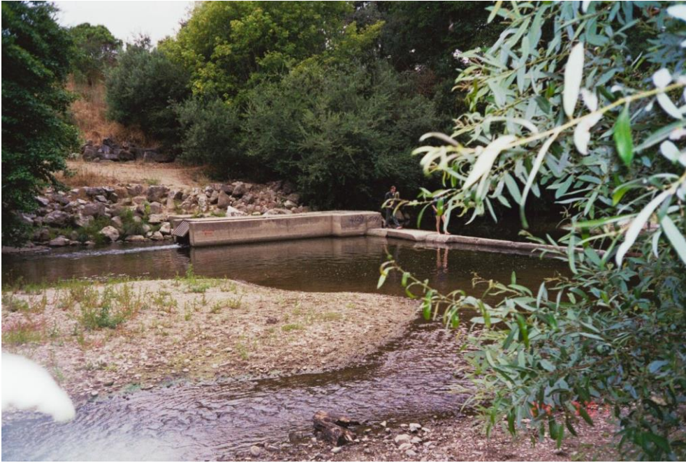
Photo: Tait Street Diversion from left bank downstream looking across the channel
