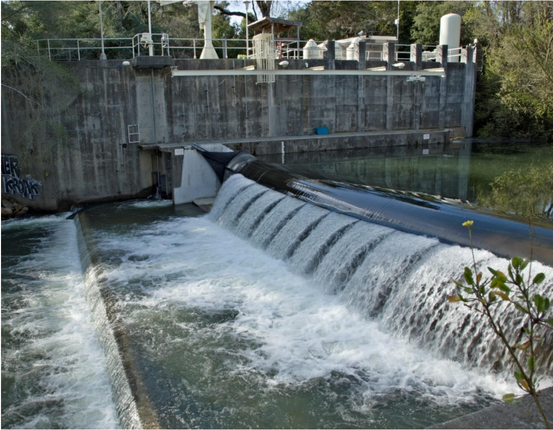
Photo: Felton Diversion from left bank downstream looking across the channel
