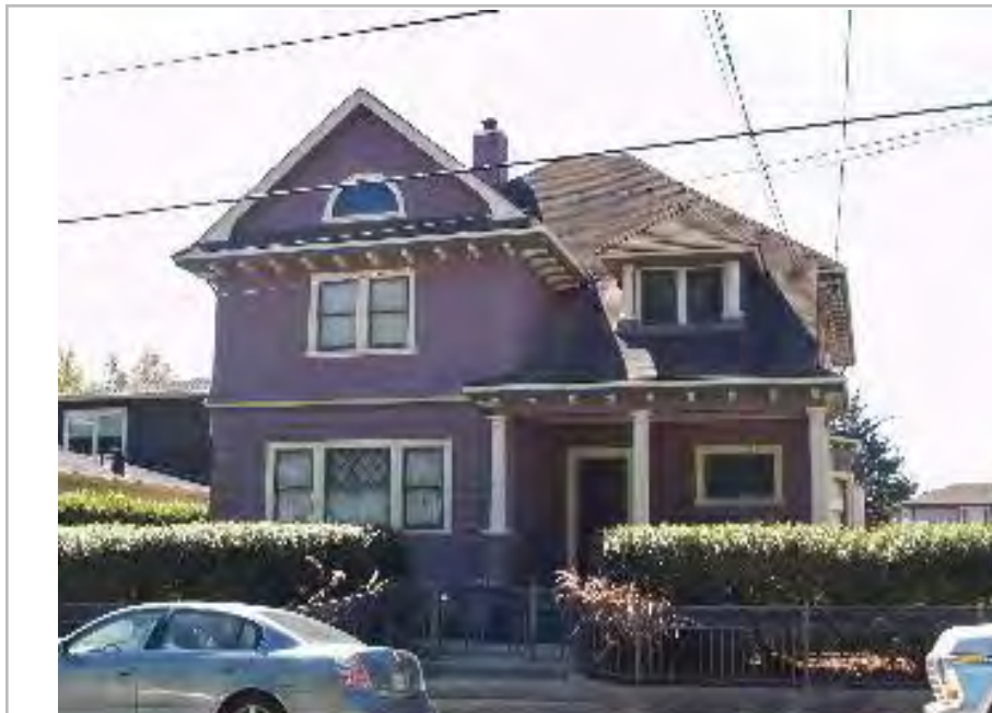
P5b. Description of Photo: (View, date, accession #) View facing south, 2009.
