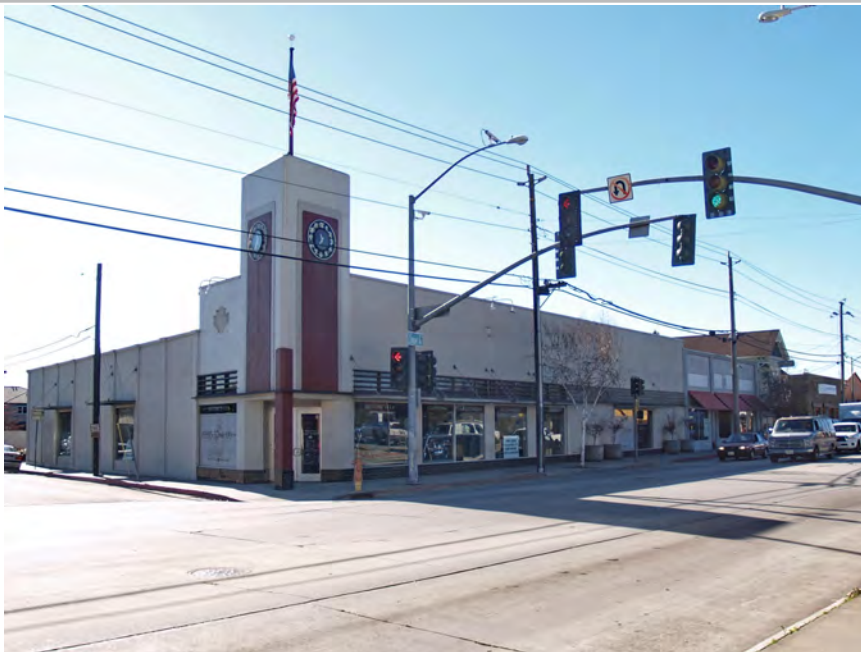
P5b. Description of Photo: (View, date, accession #) View facing northwest, 2009.
