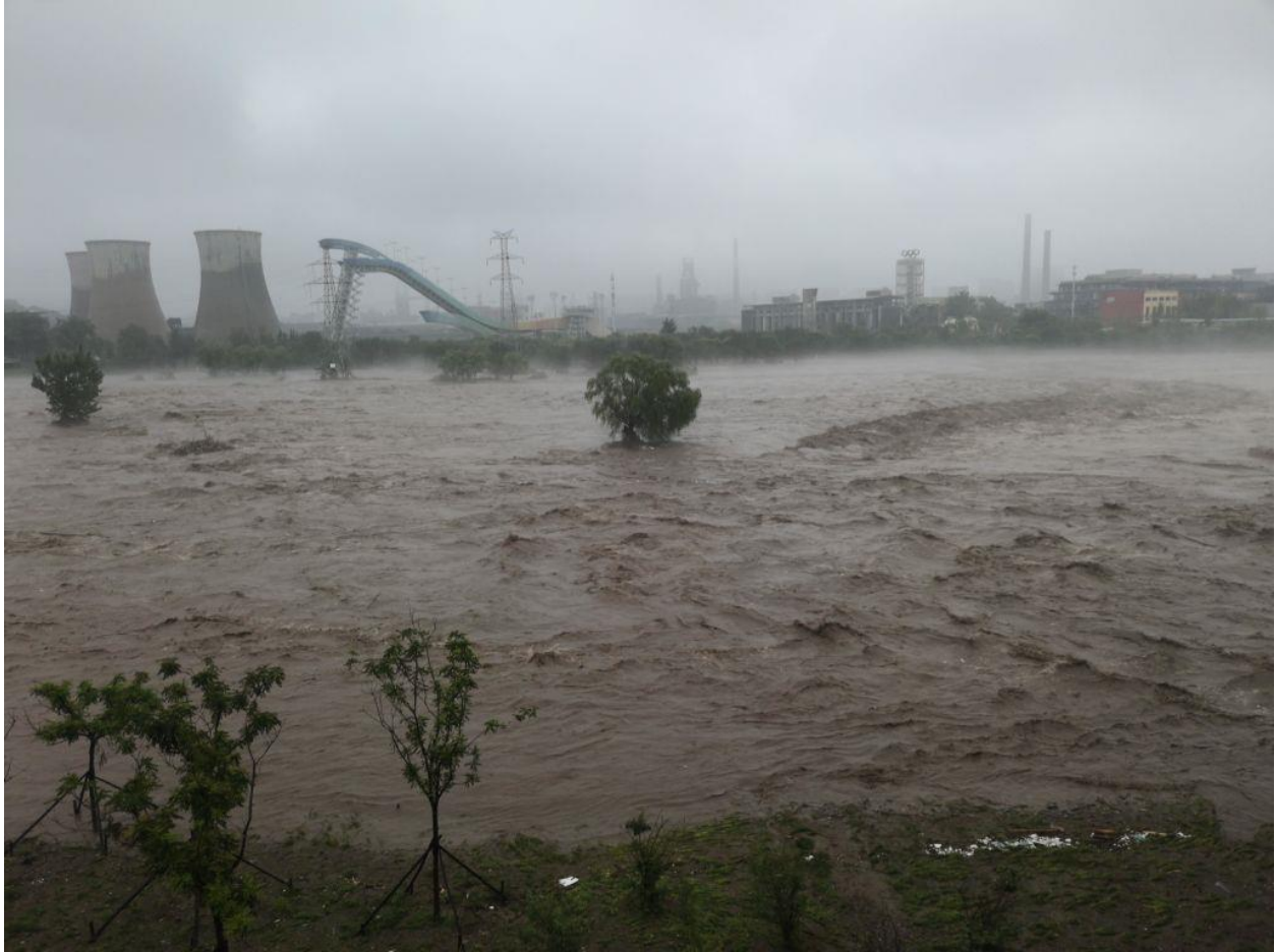
Flood waters run through the Shougang Bridge after the Yongding River was discharged in Beijing, China, August 1, 2023.
