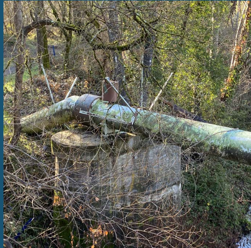
Newell Creek Pipeline Construction Manager January 2024
