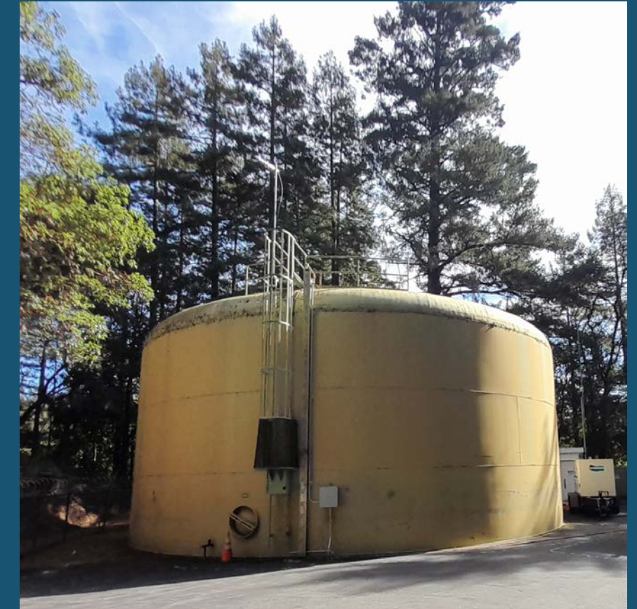
University Tank No. 4 Replacement March 2024
