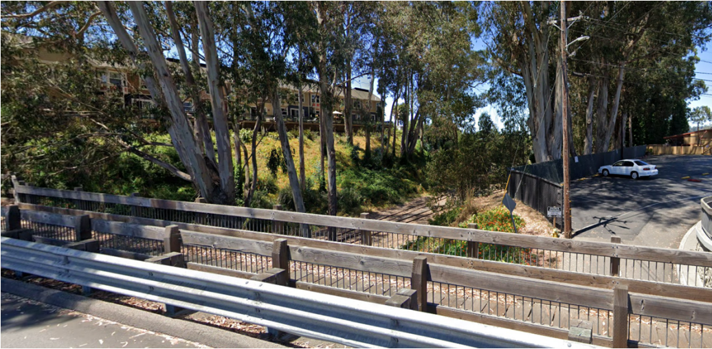
View from West Cliff Trestle
