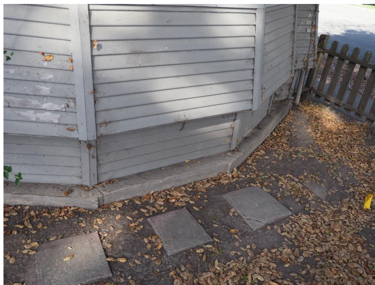
Detail view of siding at window bay
