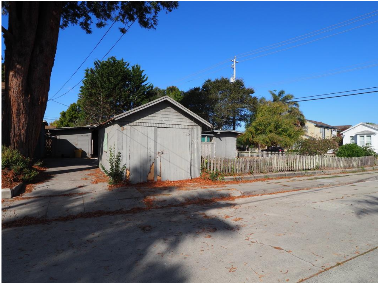
View facing northwest from 2nd Avenue showing garage and ancillary buildings
