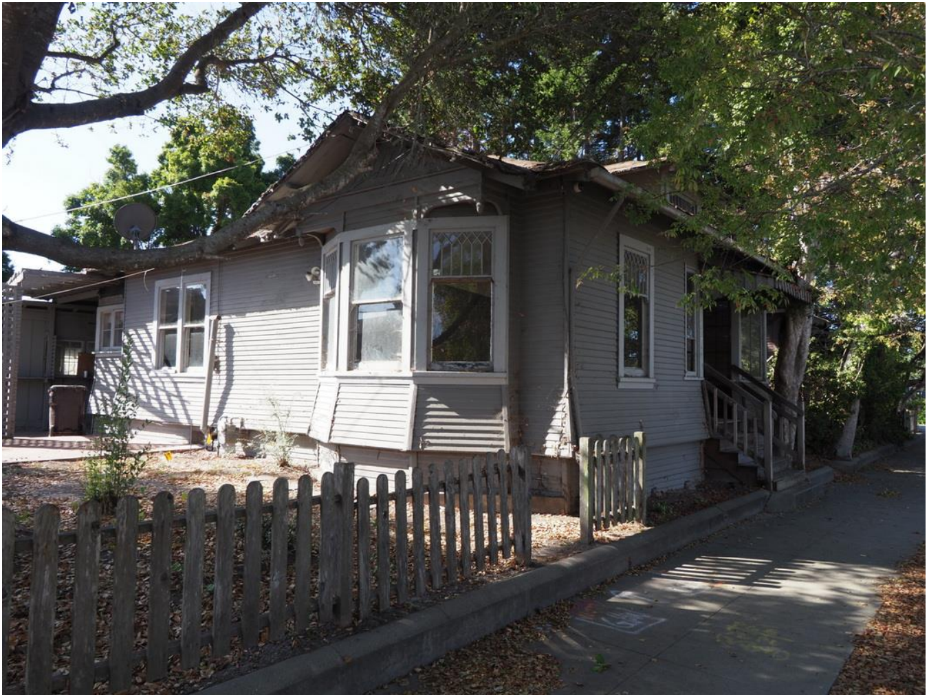
East and north (front) elevations, viewed facing southwest
