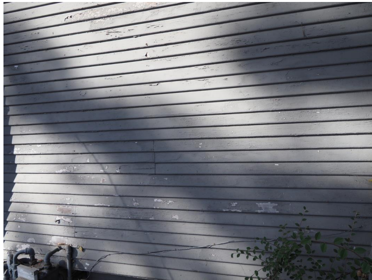
Detail view of siding
