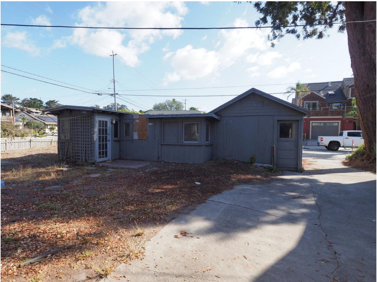
Garage and addition, viewed facing east towards 2nd Avenue
