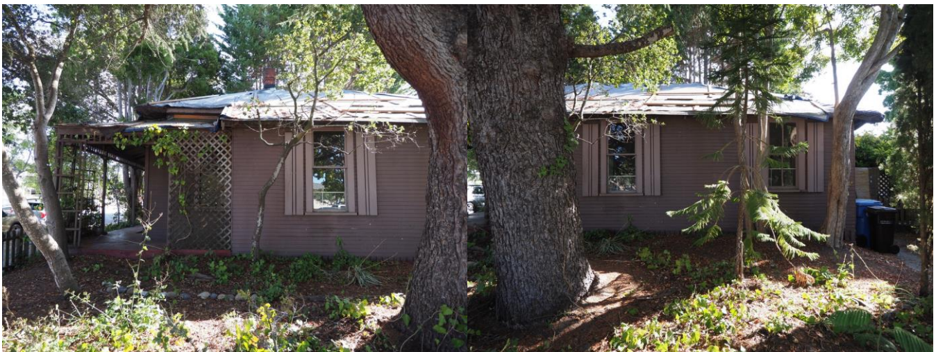
West elevation viewed facing east (composite)
