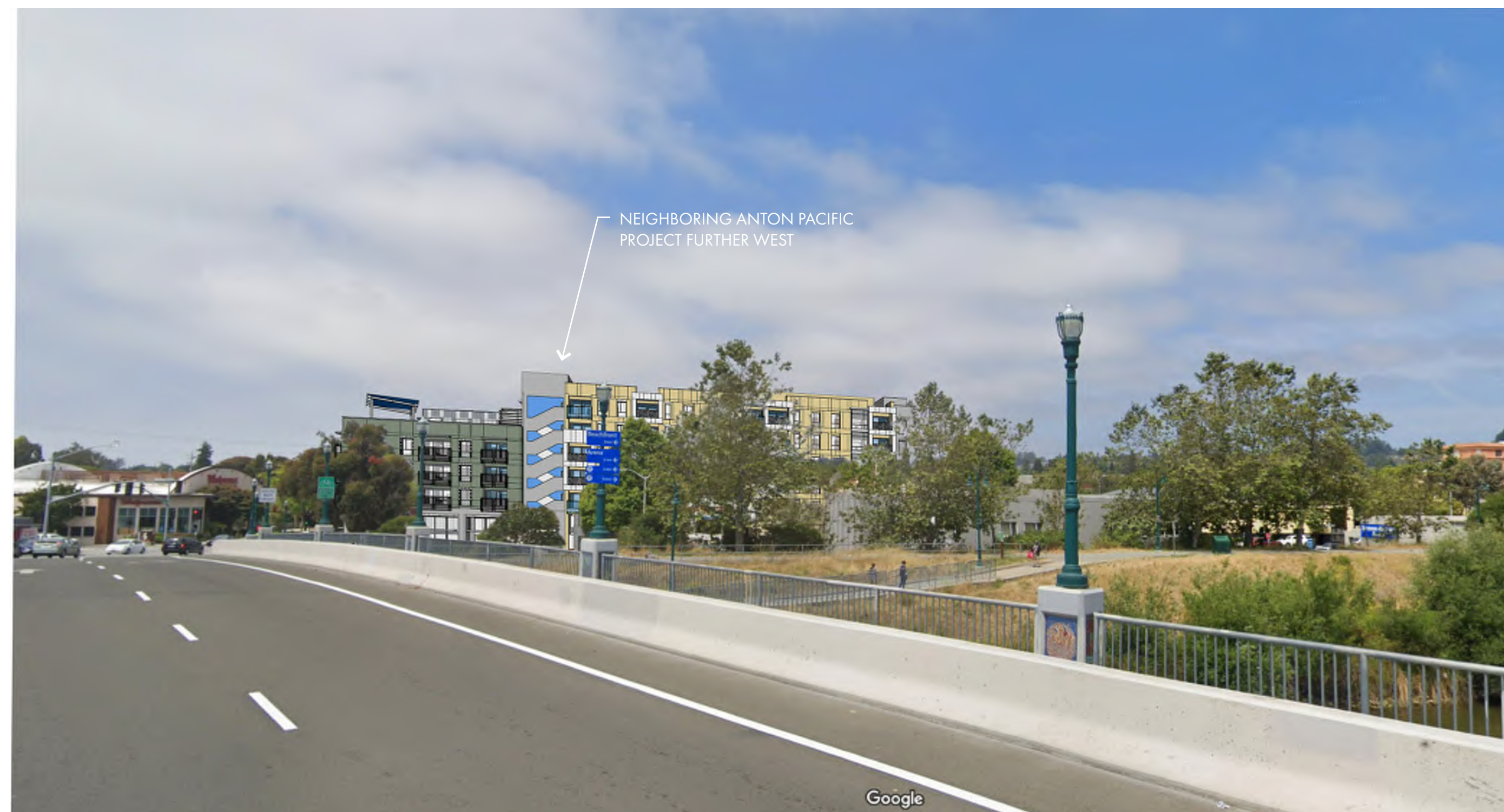
VIEW 2 (EXISTING). LOOKING NORTHWEST FROM LAUREL ST BRIDGE
