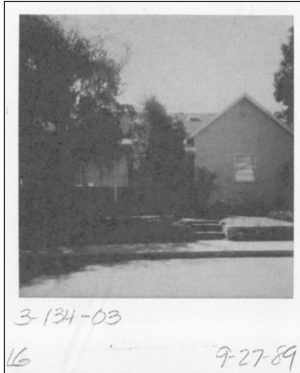
Figure 7. 1989 Santa Cruz County Assessor's image of the subject property. Note that the building was considerably altered by this date, with fenestration modified in the gable end and the front porch altered.
